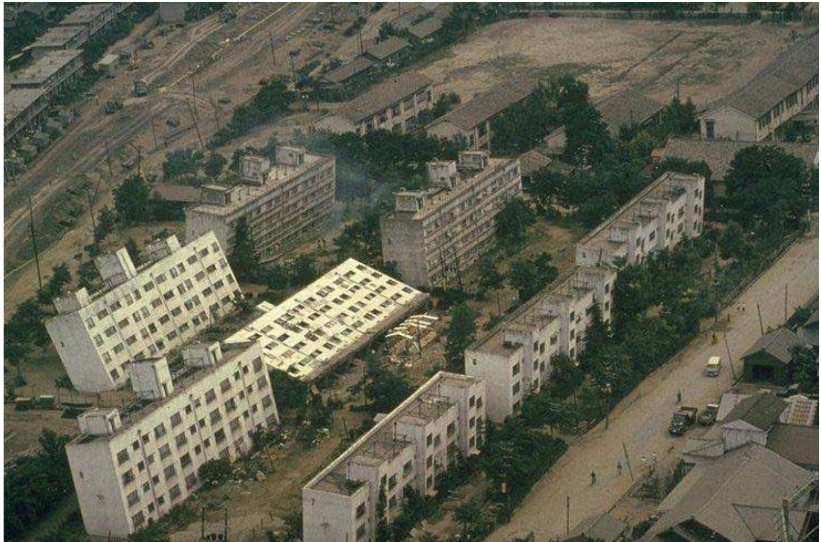
Niigata, Japan, 1964: liquefaction damage
