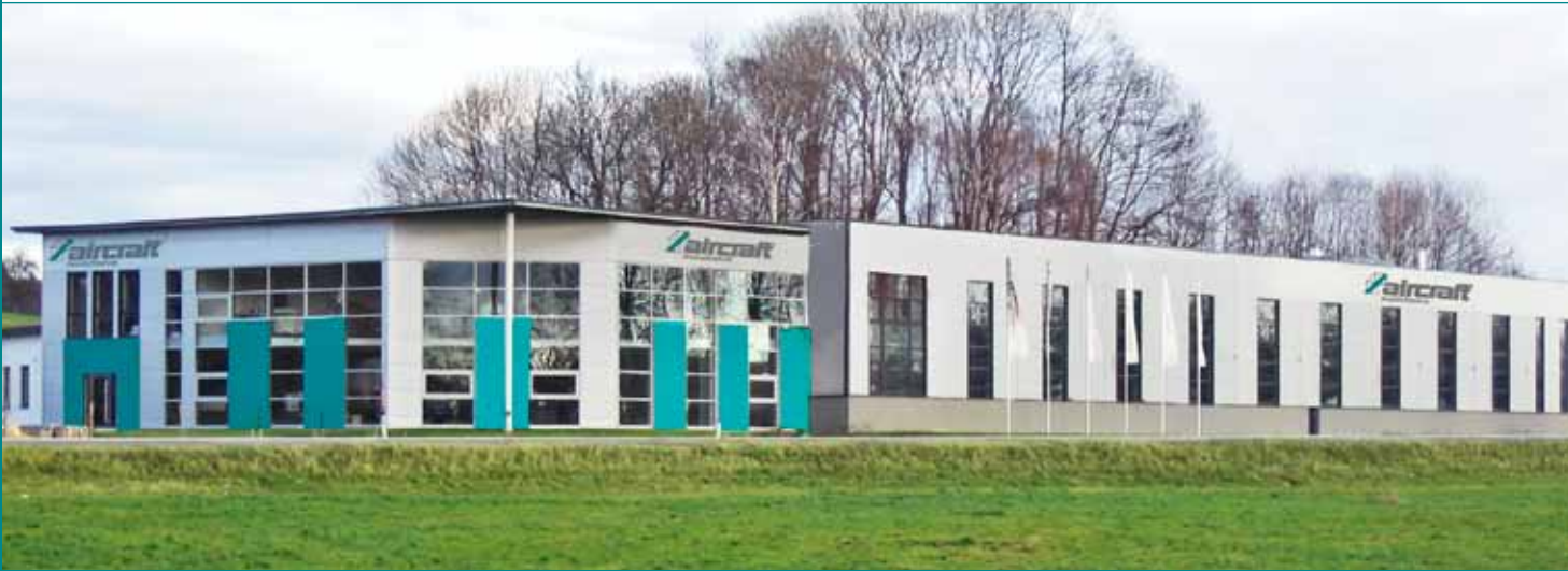
Production and administration building at Hohenzell/Austria
