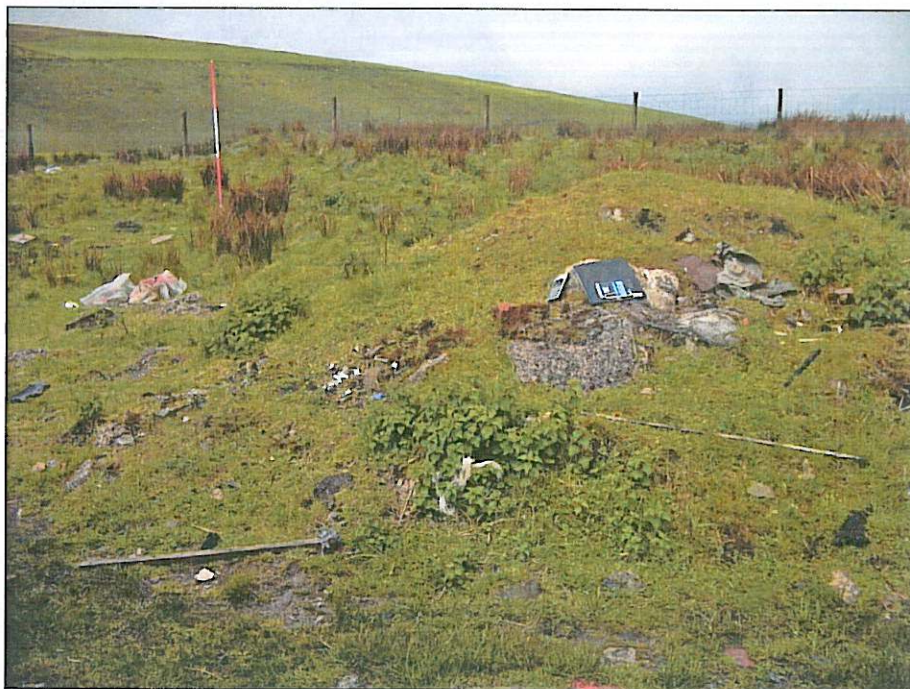
Plate 10: View to west of Bwlch Yr Afan Dyke (02265.0m) showing damaged area west of the modern track. 2m scale in shot.
