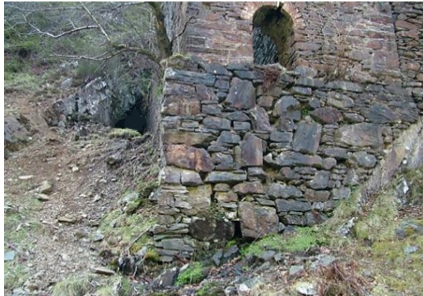
Figure 577: Temple lead mine. An adit tunnel is seen in the hillside to the left. The building on the right housed a waterwheel and ore crusher.
