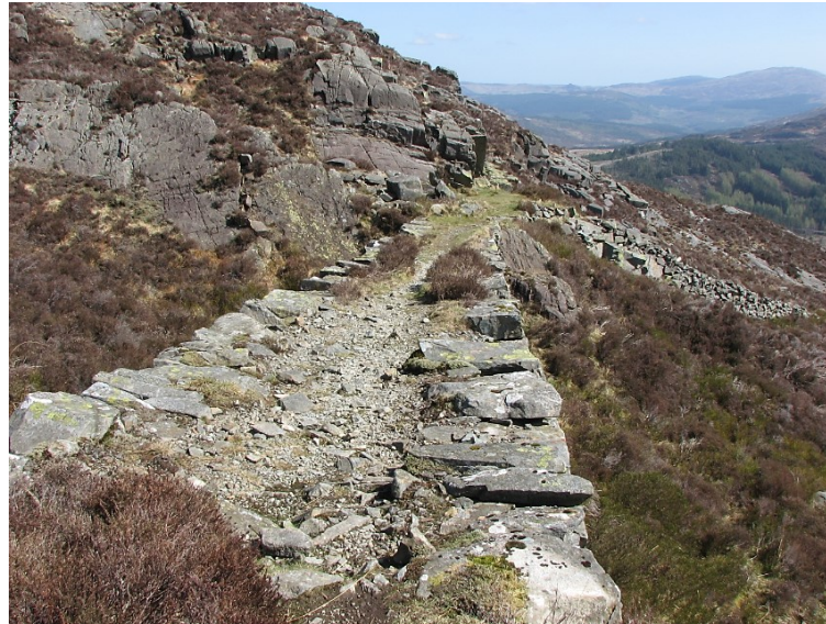
Figure 126: Tramway connecting the first and second inclines, Diffwys mine.
