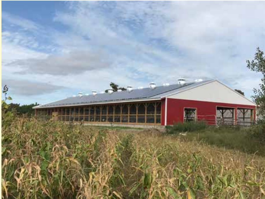
The new Sunset Lake Farm dry cow barn with its newly-installed 178kW solar PV system. Rt: The interior of the new barn in Alburgh, Vermont. Photos by Jim Merriam, Norwich Solar Technologies.
