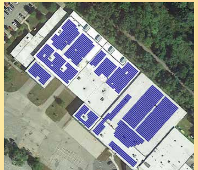
Another one of NH's largest solar arrays in Keene is 643.2kW and consists of 2,101 panels. The array is installed on the rooftops of the Keene Ice Center and adjacent Public Works Department building. Image: ReVision Energy.
