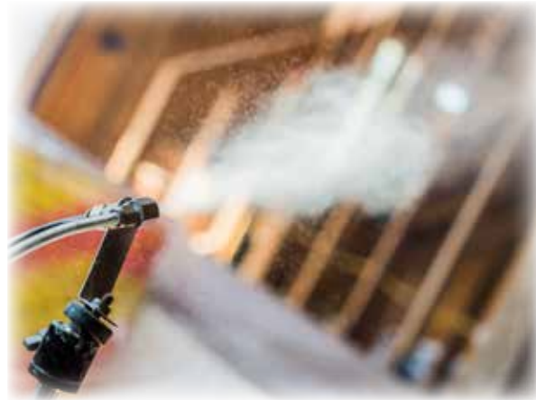
The Aerobarrier spray system in action. Photos AeroBarrier™.
