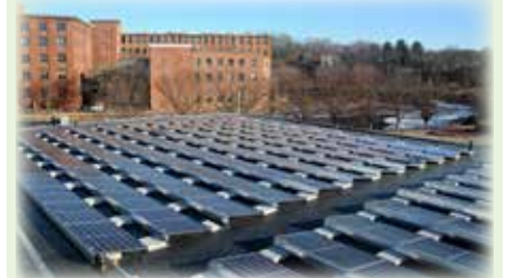
The solar array in Dover is partly installed on top of the roof of one of the town's pools, while the other is partly installed on the roof of the connecting Children's Museum of New Hampshire. Courtesy photo.
