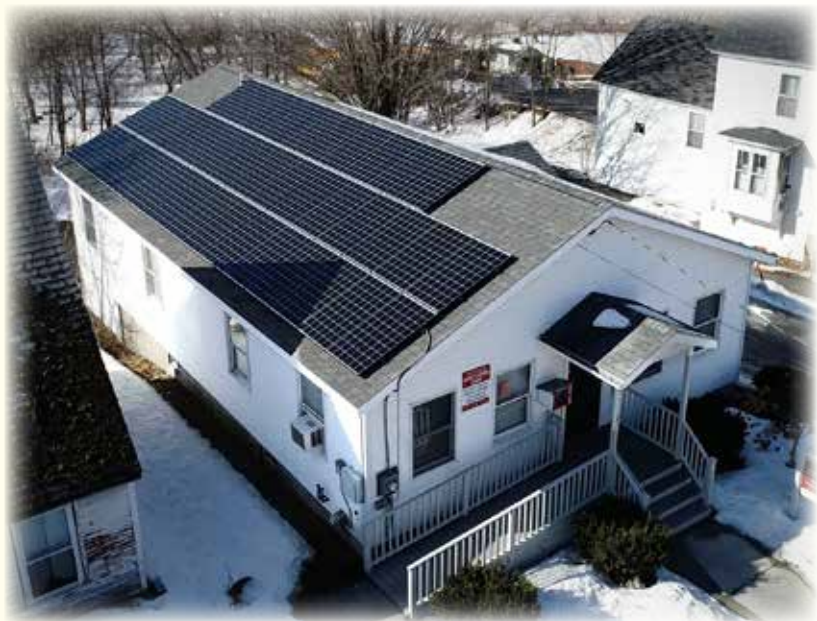
Aerial view of the Hoyt Community Care Center's 42 panel, 12.81kW photovoltaic rooftop solar array which is expected to cover 60% of its electric load. Image: Eric Rudman, Sol-Air.
