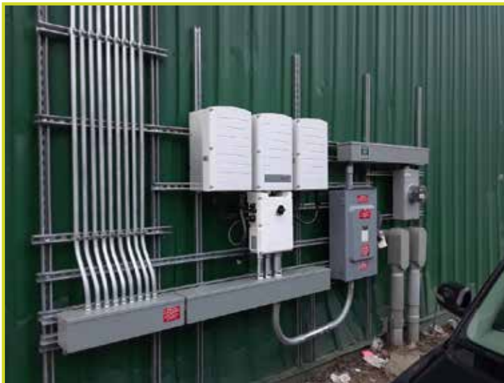
The 92kW solar array at TAM Waste and Recycling consists of array of 288 Hanwha modules, 144 SolarEdge optimizers, and one 100kW SolarEdge inverter. The system should supply 90% of TAM's electricity needs. Images: Power Guru Electric Systems
