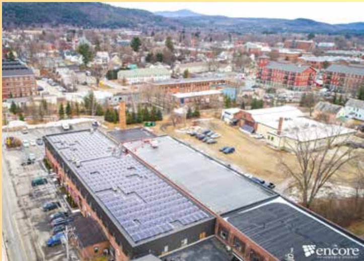
This 123.165kW DC commercial-scale roof-top solar project is located at 160 Emerald Street in Keene, New Hampshire. Image courtesy of Encore Renewables.
