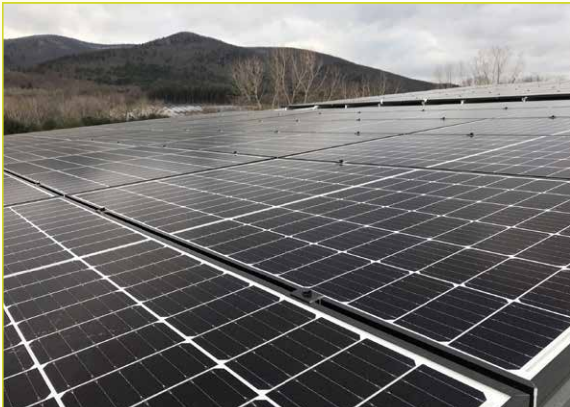
The 92kW solar array at TAM Waste and Recycling consists of array of 288 Hanwha modules, 144 SolarEdge optimizers, and one 100kW SolarEdge inverter. The system should supply 90% of TAM's electricity needs. Images: Power Guru Electric Systems
