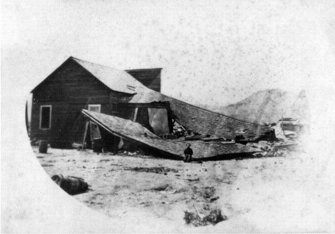
Lone Pine after the earthquake.
