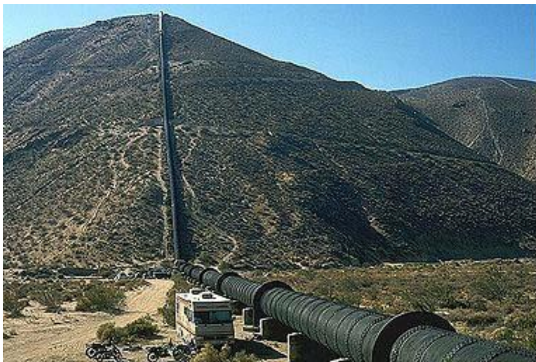
Great Siphon, LA aqueduct at Jawbone Canyon
