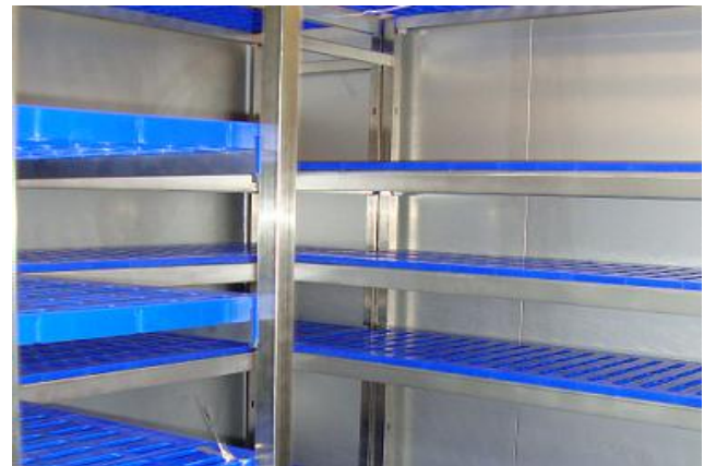
Interior shelving in stainless steel structures and polypropylene trays
