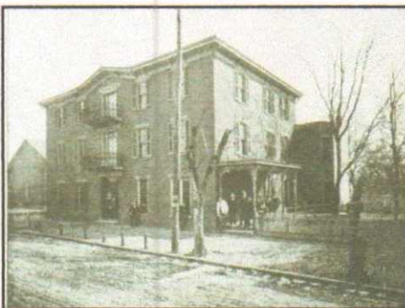
This view of the Commercial Hotel, on E. Pike St. by the railroad, is reprinted from the L&N Headlight, dated April 1898. The Civil War landmark, where Union soldiers fired from the windows at Morgan's Raiders, is still standing.
