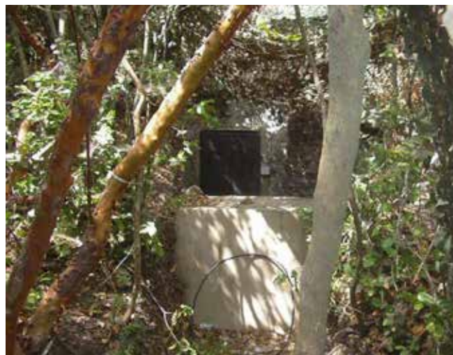
A Hizballah bunker in south Lebanon in 2006 (Credit: Israel Defense Forces)
