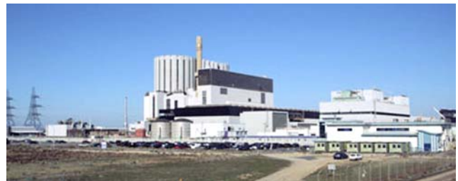
Dungeness Nuclear Power Station
