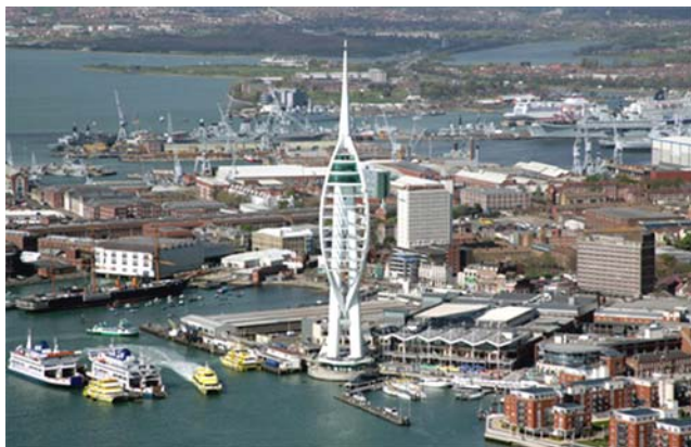
Portsmouth (Spinnaker Tower)
