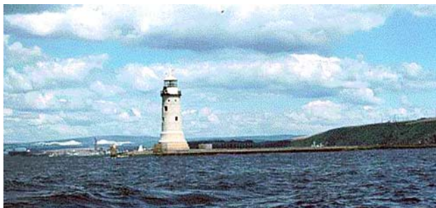
Plymouth Breakwater West Light
