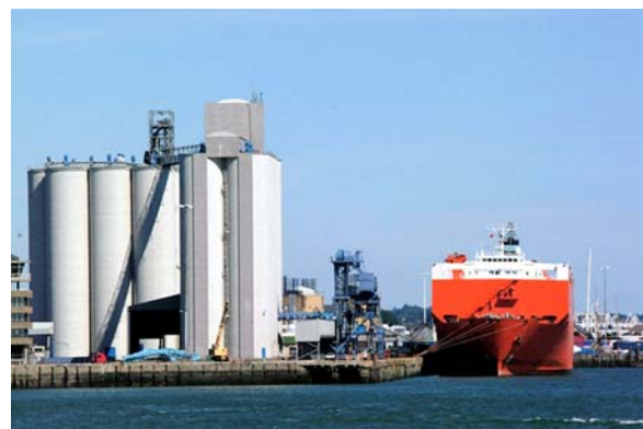
Eastern Docks Silo
