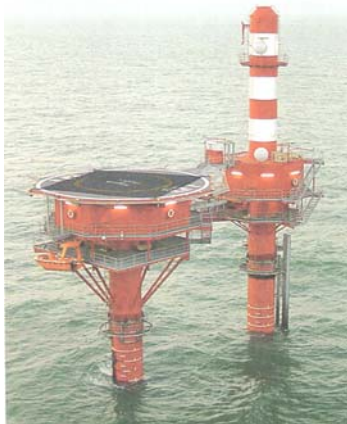
Oost Dyck Radar Tower
