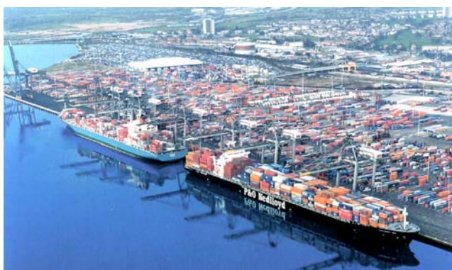
Southampton Container Terminal
