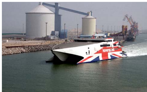
High-speed ferry passing bulk berth silos
