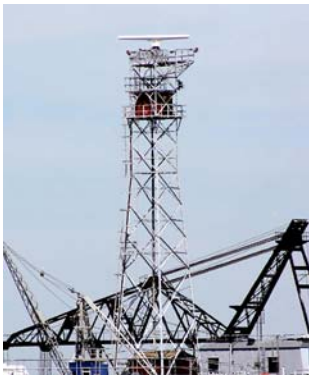
Admiralty Jetty Radar Tower
