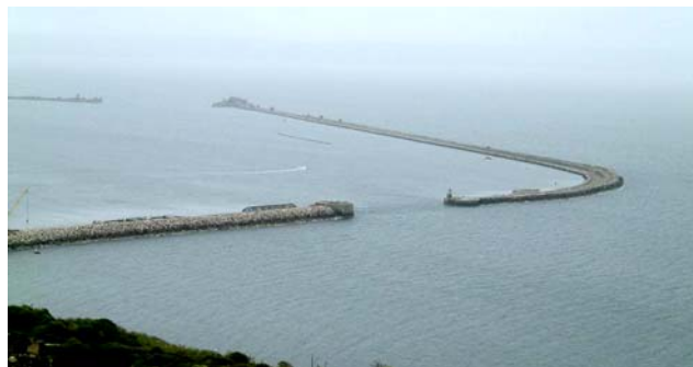
Portland Harbour Breakwaters
