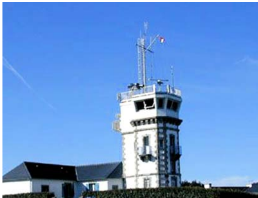
Ile de Brehat Signal Station
