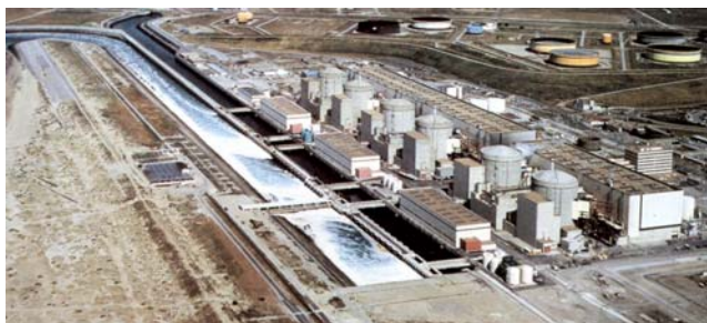
Gravelines Nuclear Power Station
