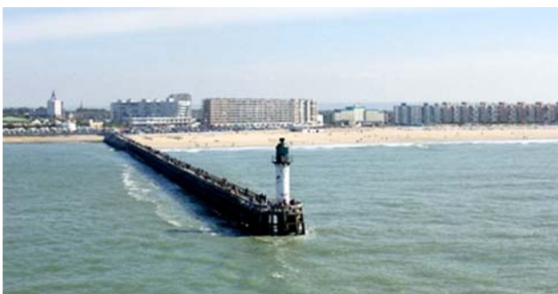
Calais West Jetty Light
