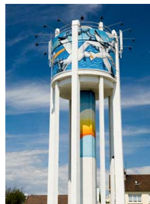
Calais—Bleriot-Plage water tower
