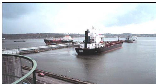
Goteborg—Sarvik Oil Terminal
