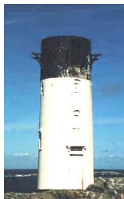
Ursholmen Disused Light Tower
