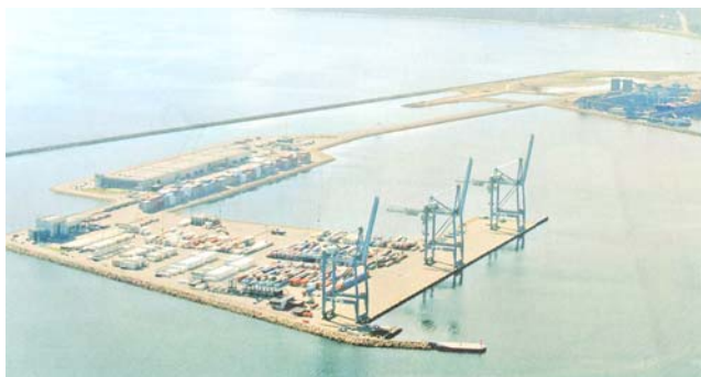
Arhus—New container terminal
