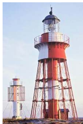
Maseskar Light (background) and Disused Light Tower
