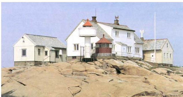
Stromtangen Light (with disused lighthouse)
