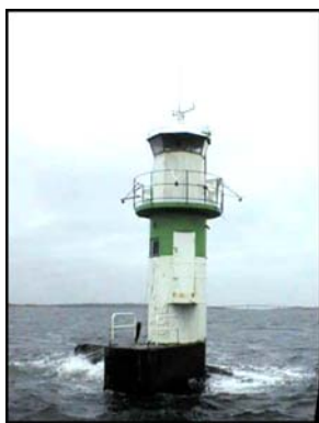
Mavholmsbaden Disused Light Tower (Racon)
