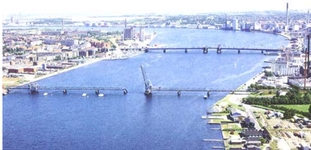
Aalborg—Bridges from W
