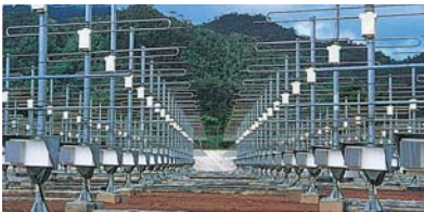
Equatorial Atmosphere Radar in West Sumatra, Indonesia. Its size is about the same as that of an MU radar.
