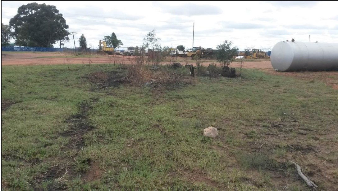
Figure 5: Representative photograph of the transformed habitat unit around Alternative 1.
