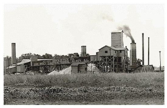
Figure 2. Circa 1910 photograph of the Alsey Brick and Tile Company on the southeast edge of Alsey, Illinois (Alsey Refractories Company website, July 2005 [http://www.alsey.com/history 06-49.htm]). Among the various structures visible in this image are several beehive kilns, primarily visible by their chimneys, and what appears to be a mineshaft and tipple complex.
