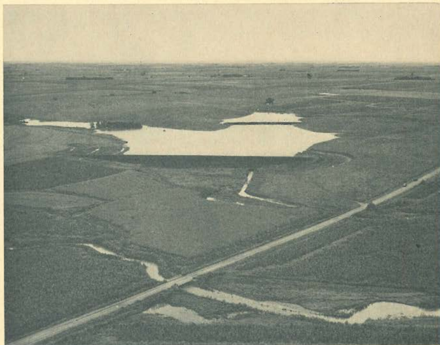
Below: Floodwaters are released slowly through 18-inch "trickle pipe" into the creek below this dam.
