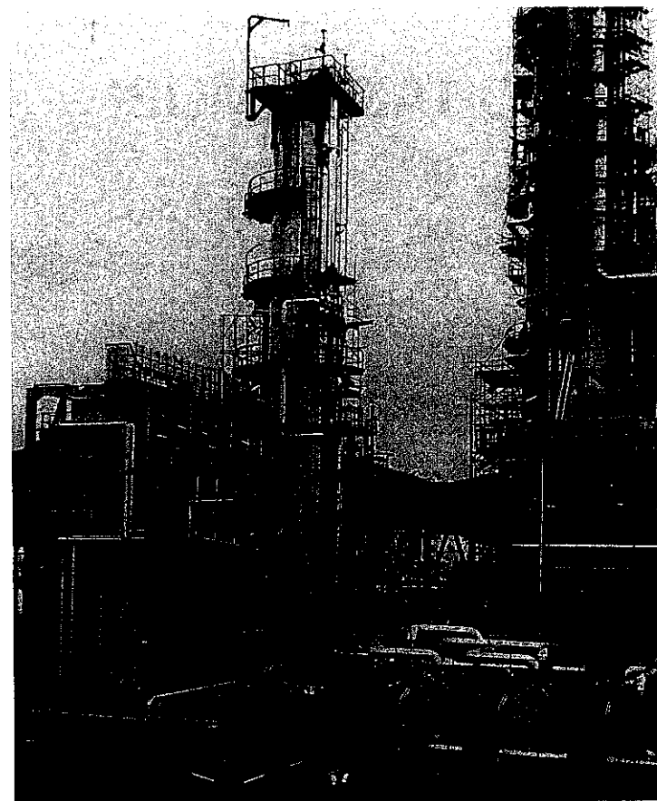
FIGURE 8.7.4 Exxon-designed Hydrofiner treating mixed virgin/cracked stock to stringent sulfur specifications in Southeast Asia.
