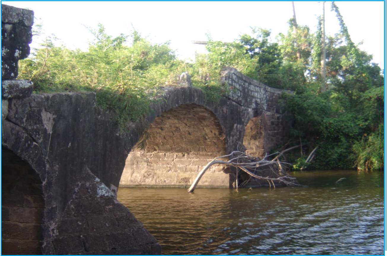
Photo 3.0. Big Creek Bridge (photo Lucia Mings).
