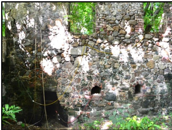
Photo 121. The furnace's stoke holes with the "fatch" furnace to the left, Brewer's Bay Sugar Works.
