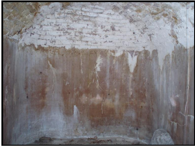
Photo 97. Interior of the cistern at Fort Charlotte.
