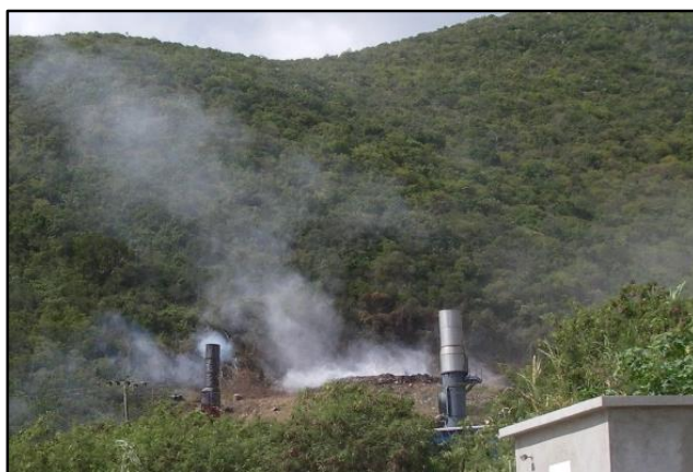
Photo 142. The incinerator at Pockwood Pond, Tortola.
