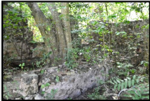
Photo 118. The copper battery inside the boiling house, Brewer's Bay Sugar Works.
