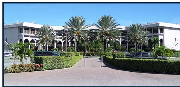
Photo 15. Government Administration Building, Road Town.
