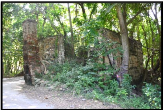
Photo 116. The boiling house at Brewer's Bay.
