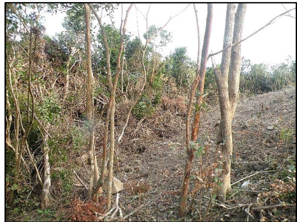
Photo 154. Right half of photo shows land recently cleared of vegetation by a bulldozer, along a steep slope on Tortola. Exposed soils are vulnerable to erosion.
