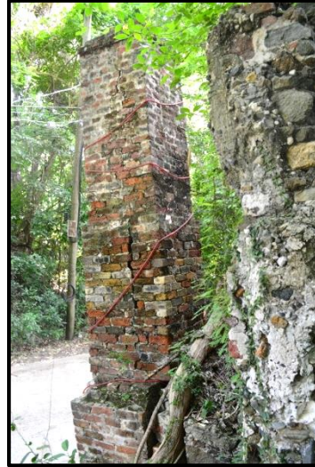
Photo 120. Red-brick chimney at Brewer's Bay.
