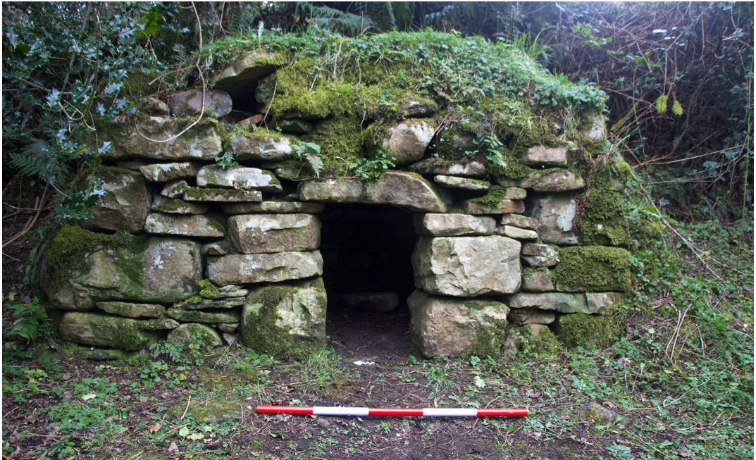
Figure 1. Exterior view of the sweathouse at Cleighran More, County Leitrim (SMR no.: LE020-005). This sweat-house is roughly D-shaped, has a lintelled roof and the entrance faces west. A seating stone is visible within the interior. This structure was conserved during the 1980s and it is situated in a public amenity area. This structure is only marked on the 6-inch Ordnance Survey (OS) maps. Photograph by Katie Kearns, 2020.
