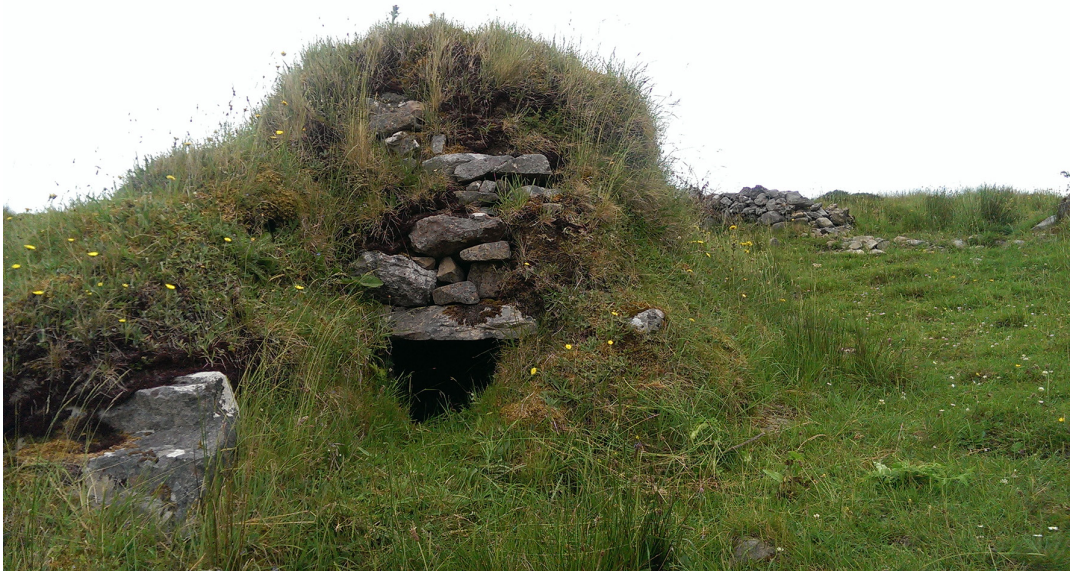
Figure 5. The free-standing sweathouse at Legeelan, County Cavan (SMR no.: CV004-011). The south-west facing entrance is made narrower by an accumulation of earthen deposits. The chamber is beehive shaped and is roofed by a single slab in the interior. This sweathouse is marked on the 25-inch and 6-inch Cassini OS maps. Photograph by Katie Kearns, 2016.
