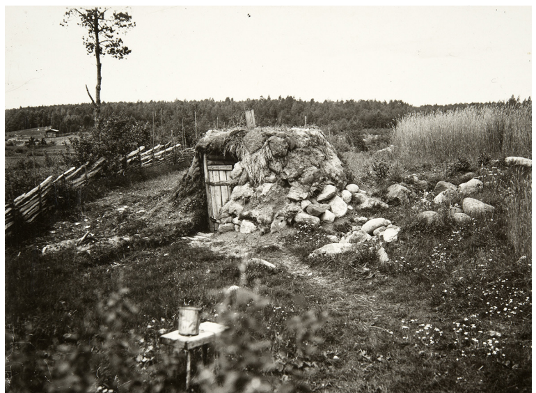
Figure 6. Finnish maasauna covered by an earthen layer. Photograph by Eino Nikkilä, 1931, Finnish Heritage (Museovirasto).
