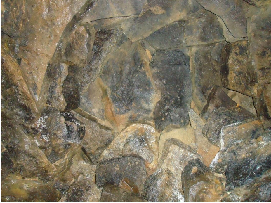
Plate 15. The interior corbelled roof of Coppanaghbane sweathouse, Co. Cavan (image by the author).
