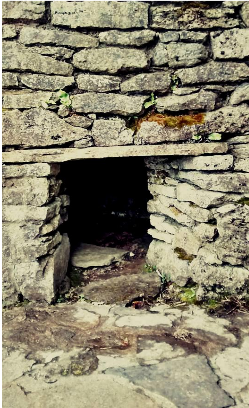
Plate 8. View of the south-west facing lintelled entrance of the restored sweathouse at Kilmore, Co. Leitrim. This is on the site of Parke's castle, a national monument in State care. (Image by the author).
