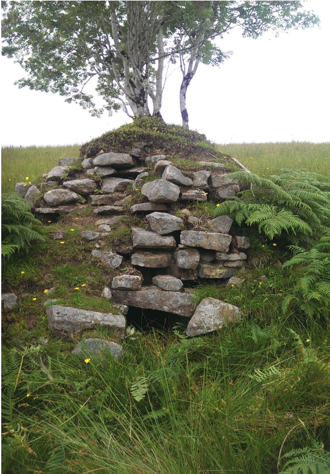
Plate 3. The conical shaped mound of the sweathouse at Gubnaveagh A, built into a slope which is visible in the background. The east-facing lintelled entrance is considerably low. Gaps in the stonework above the entrance and on the top right may have allowed smoke to escape in the stead of a chimney hole. Growing on top of the structure is a young mountain ash tree (image taken by the author).
