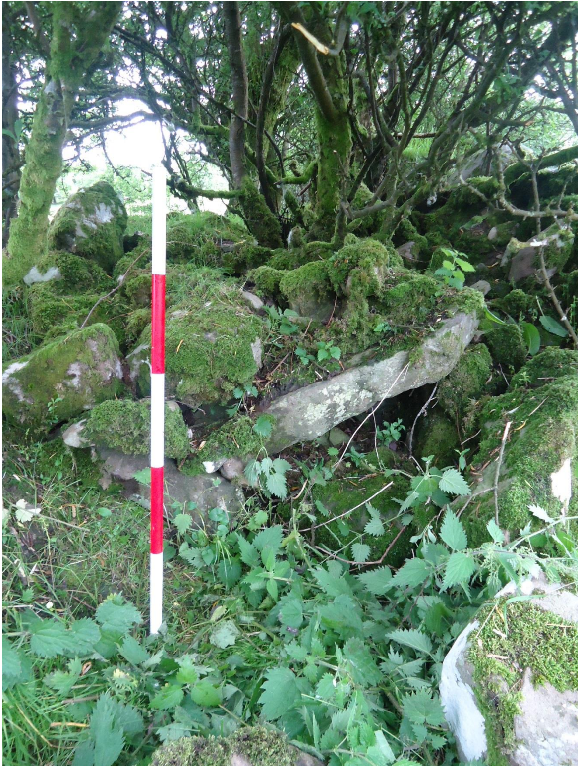
Plate 2. The collapsed east-facing entrance of the sweathouse at Lisgorman, Co. Leitrim. The possible entrance lintel is still visible in the centre right of the photograph. Tree and vegetation growth have contributed to the deterioration of this structure (image taken by the author).
