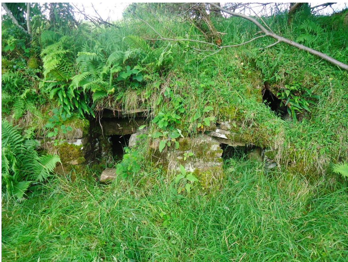
Plate 5. The partially collapsed, overgrown double-chambered sweathouse(s) at Crosshill, Co. Roscommon. The roof and entrance have collapsed in on the eastern chamber. The western chamber is intact, but is structurally vulnerable. Both south-facing entrances are lintelled (image by the author).
