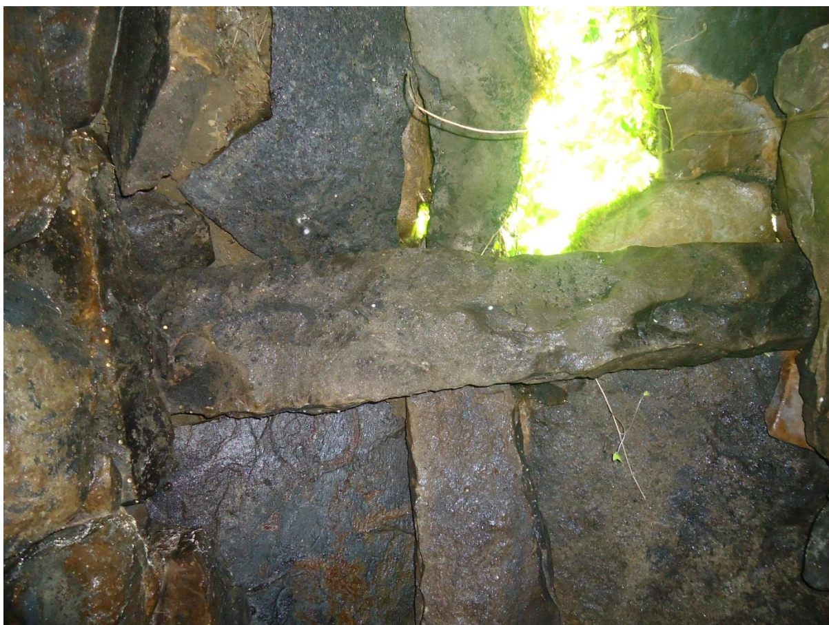
Plate 12. An interior view of the lintelled roof of the sweathouse at Cleighran More, Co. Leitrim (image by the author).
