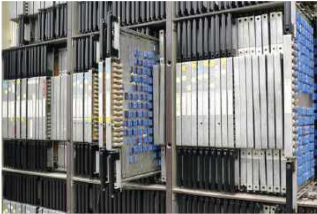
Boards from the ILLIAC 4 computer, state of the art in 1966.
