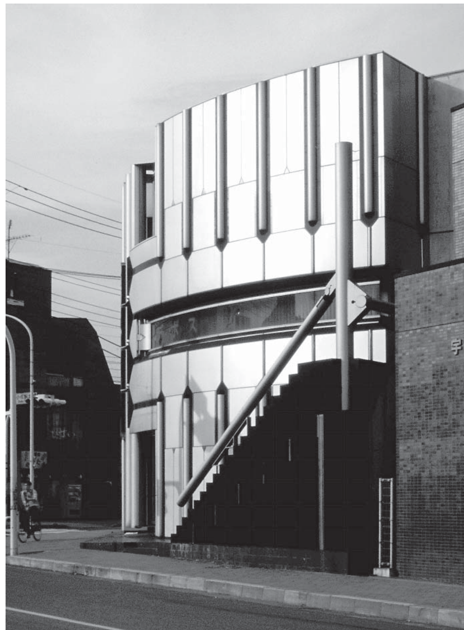
Shin Takamatsu: Wako Headquarters Building, Ome, Tokyo (1989)
