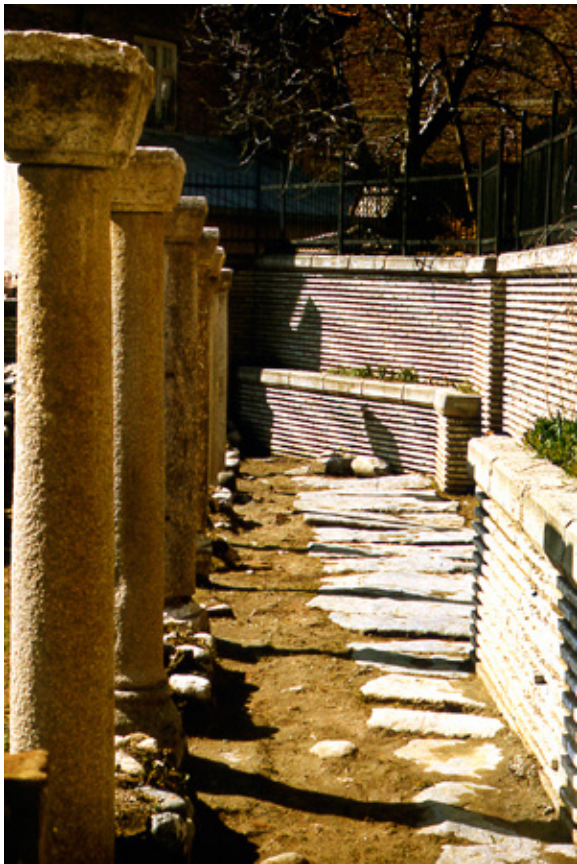
Fig. 14. Anastylis of the Eastern colonnade on Via Sacra / Mese. Marble and granite bases, bases-postaments and columns.
