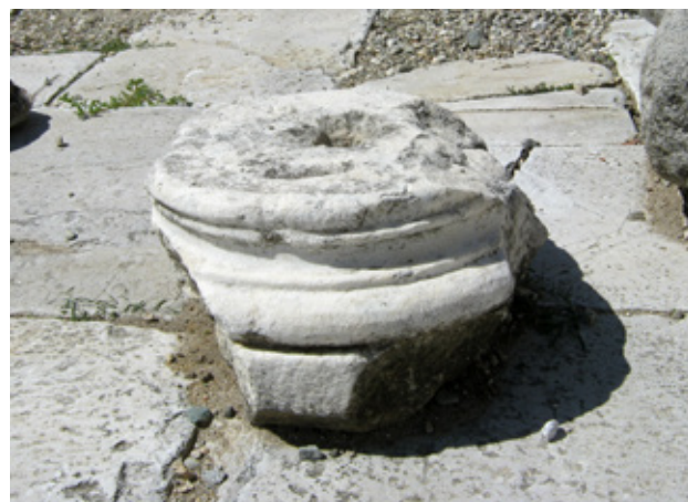
Fig.5. A marble Attic-Ionian base: two toruses, trochilos and two listels from basilica No 1.
