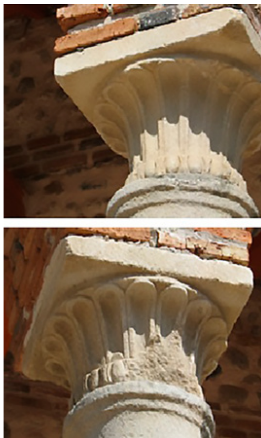
Fig. 21. Marble Roman-Dorian capitals, type II, variant B. The Northern colonnade in the atrium of the Episcopal basilica.
