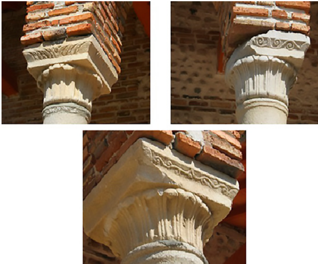
Fig.20. Marble Roman-Dorian capitals of type II, variant A, with compound profiled abacus. The Northern colonnade in the atrium of the Episcopal basilica.
