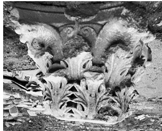
Fig.33. A marble Roman-Corinthian column capital. The colonnade of the naos in the Episcopal basilica, first floor.
