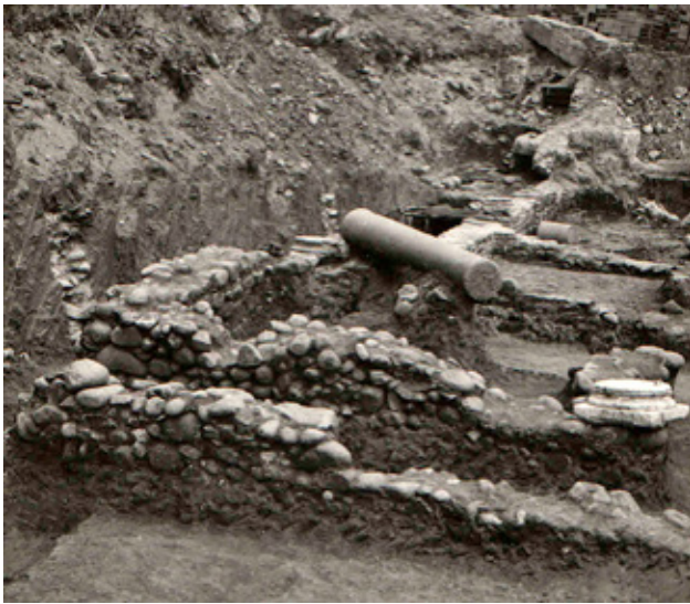
Fig. 2. The Roman and the Late Roman building under GUM, view from southwest (photo of V. Popova).
