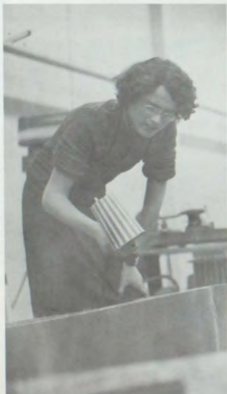
Donald Struthers applies the final layers of fibre glass to a boat.
