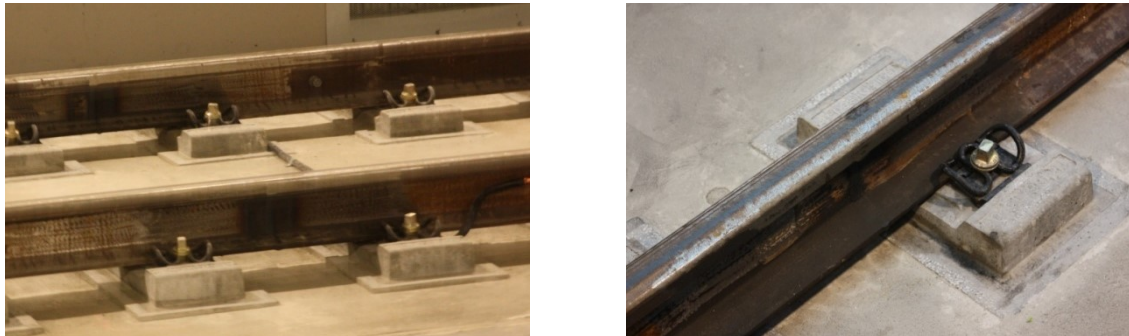
Picture 8 Thermite weld: a). Side view; b). Overview Source: Own archive
