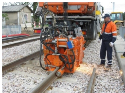
Picture 4. Flash-butt welding machines: a). stationary, b). two-way machine type KCM-005 (source: own archive and https://torpol.pl )
