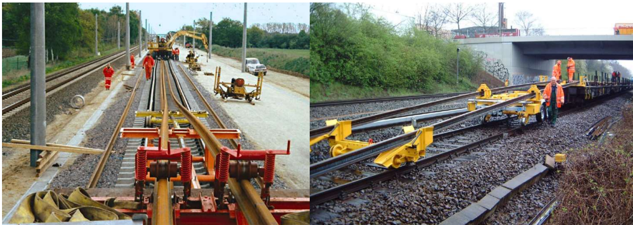
Picture 6. a). Last platform equipped with special devices expediting the unloading process; b). Special devices expediting the unloading process located out of the platform (source: a). http://www.vossloh-rail-services.com ; b). http://cemafer.com )
