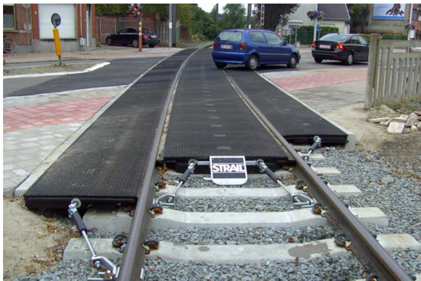
Fig. 3. Pontistrail type surface on level crossing in Belgium (Strail www-site)
