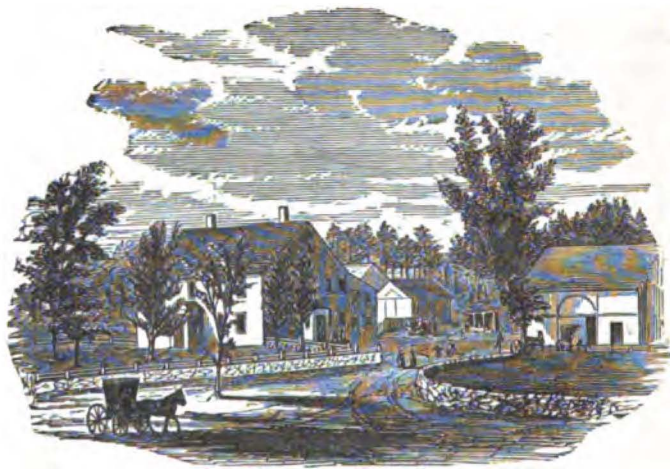
RESIDENCE OF MR. MARTIN STETSON.
