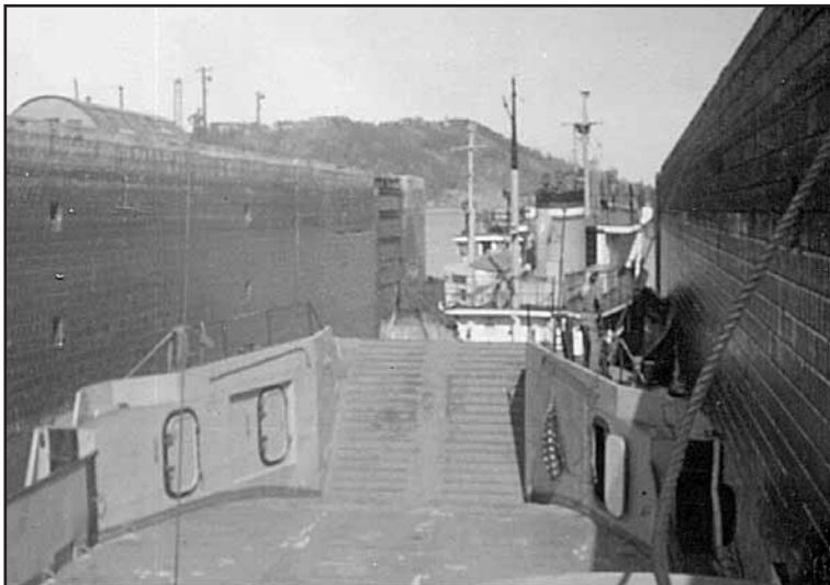
One of the docks the 18th Heavy Boat Company used to offload troops and supplies
