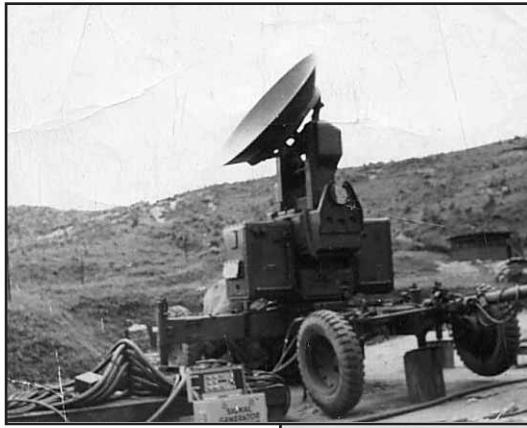
At left, The counter mortar radar and, below, the installation at "Charlie Block" near Munsan-Ni
