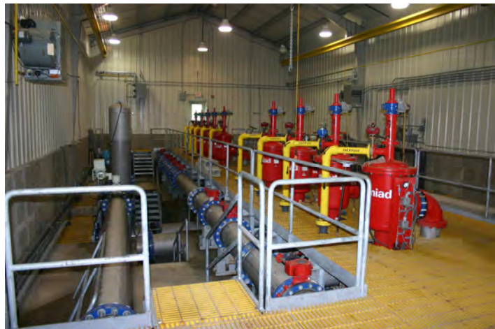
Figure V-4. Pressure Strainer Array
