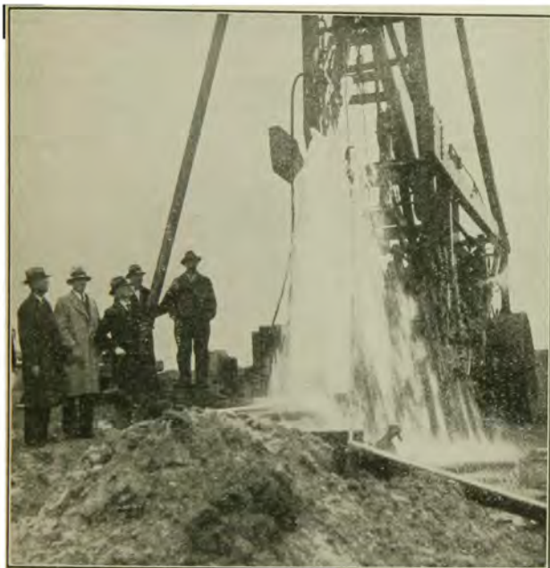
Figure 10. EAST ROCHESTER ARTESIAN WELL, NO. 1 Preliminary test, November 8, 1934
