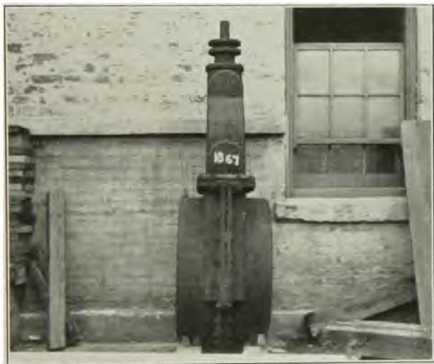
Figure 1. IRON GATE Intended for use in the wooden conduit. 24-inch
