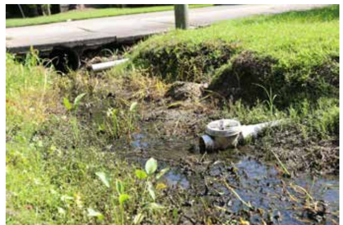
Septic ditch. Photo by Jennifer Bushnell
