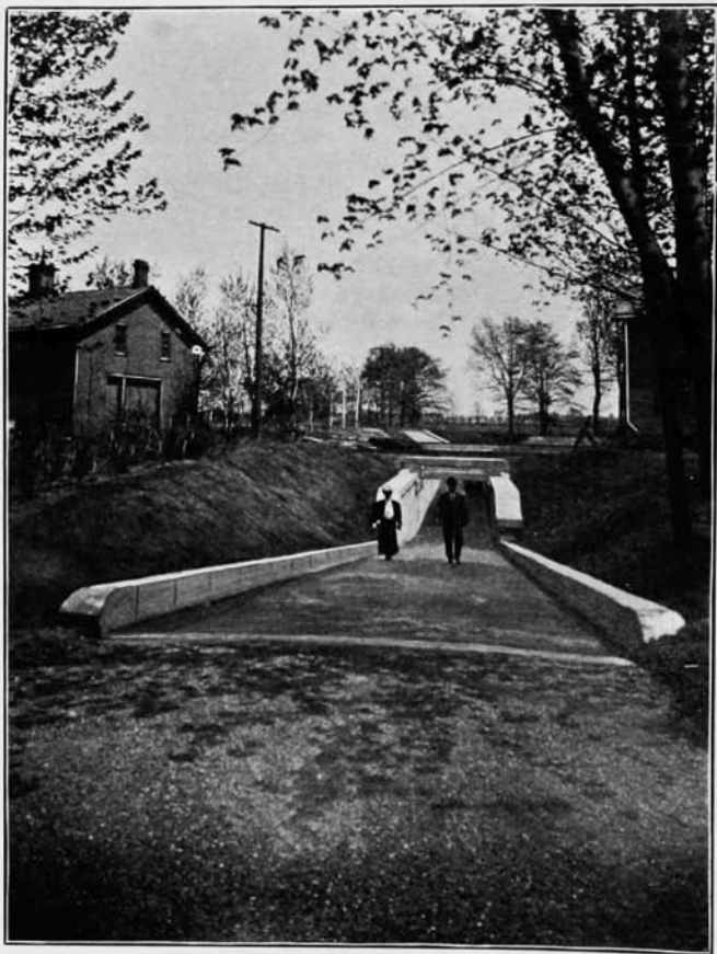
Subway—Genesee Valley Park
