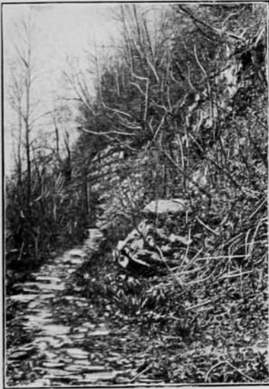
Buell Avenue, Spring 1905 -Maplewood Pk.
