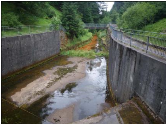
Plate 8.7: Altnaheglish Dam outfall
