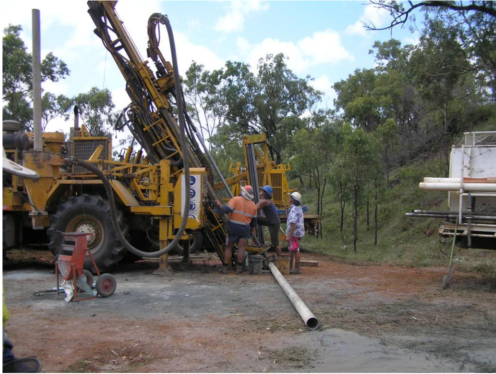
Figure 19 - Drill rig on site of IGRC002, looking south. Cyclone and sample splitter in left of photo (Terra Search, 2011)
