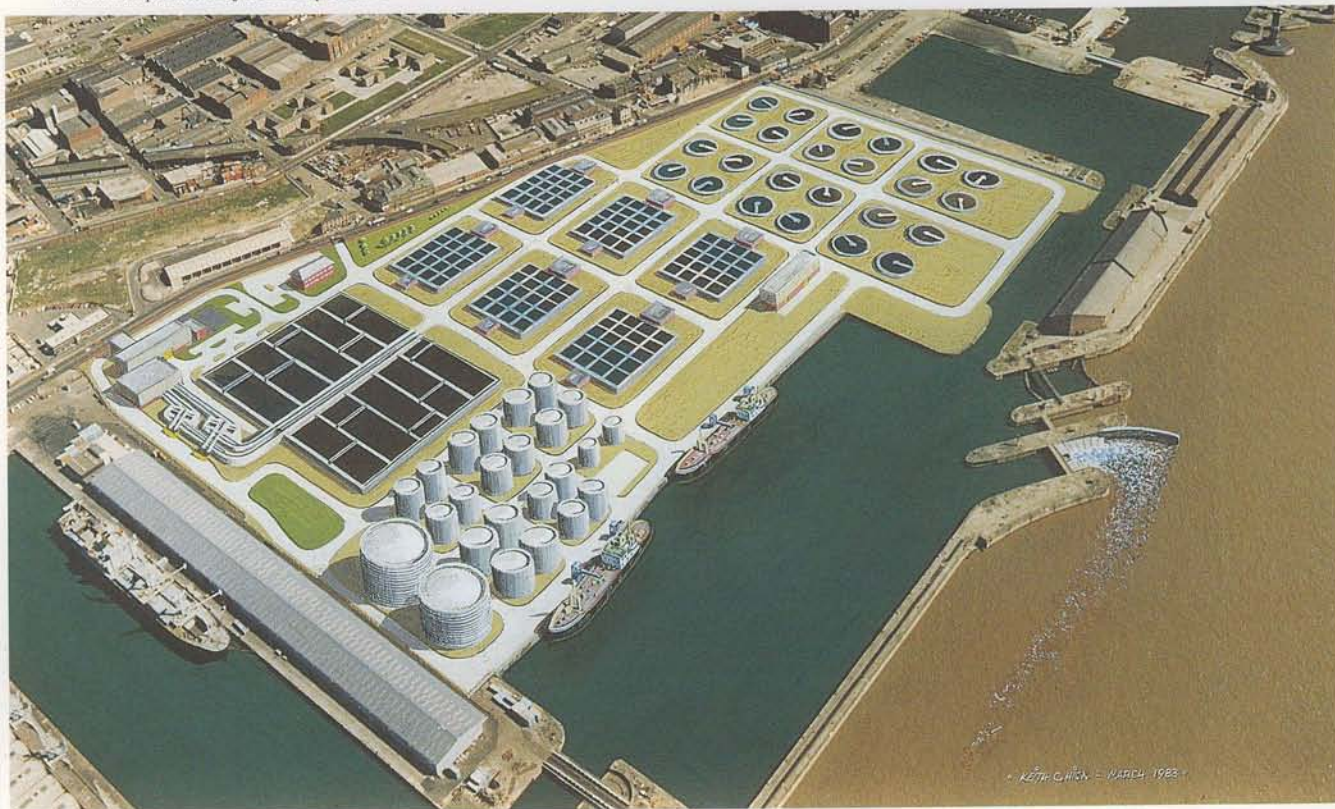
Artist's impression of the completed Sandon Dock Wastewater Treatment Works.
