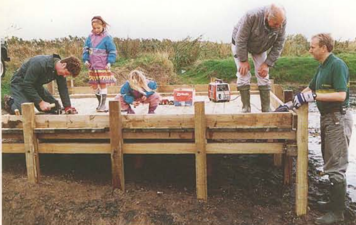
Building a dipping platform thanks to a Waterside Revival grant
