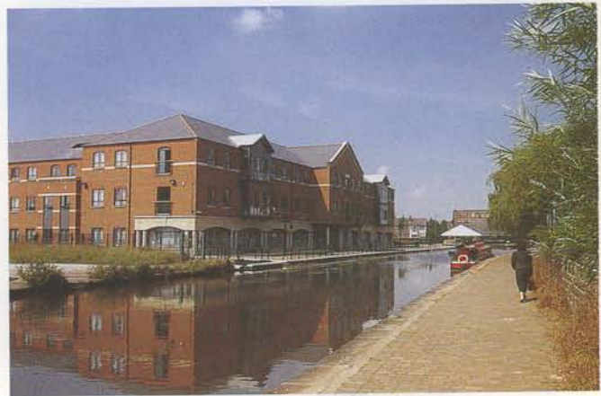
Leeds - Liverpool Canal at Wigan Pier
