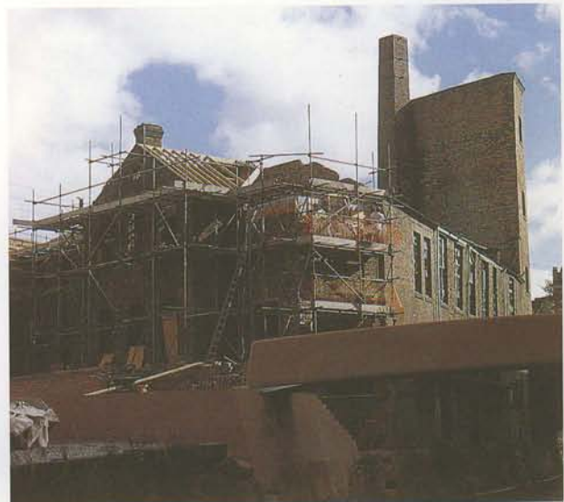
Renovating a derelict warehouse at Castlefield, Manchester
