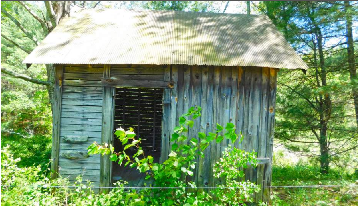
A. East Facing Side of Crib
