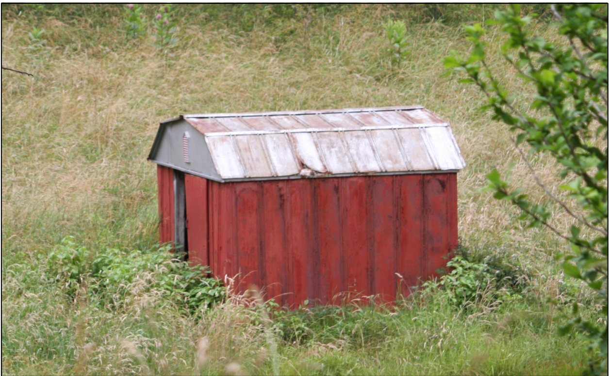
Figure 12. 035-5136, Metal Shed. Photo taken 23 June 2017, facing east.
