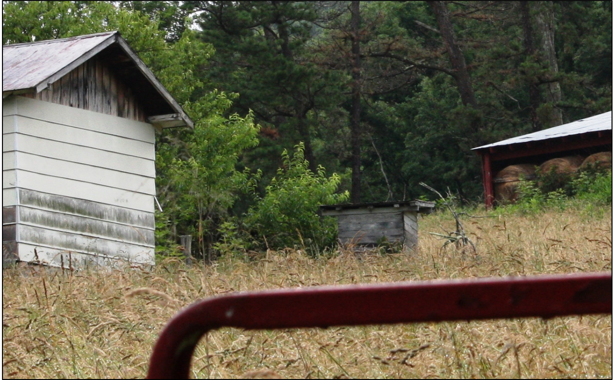
Figure 13. 035-5136, Small Wood Building. Photo taken 23 June 2017, facing west.
