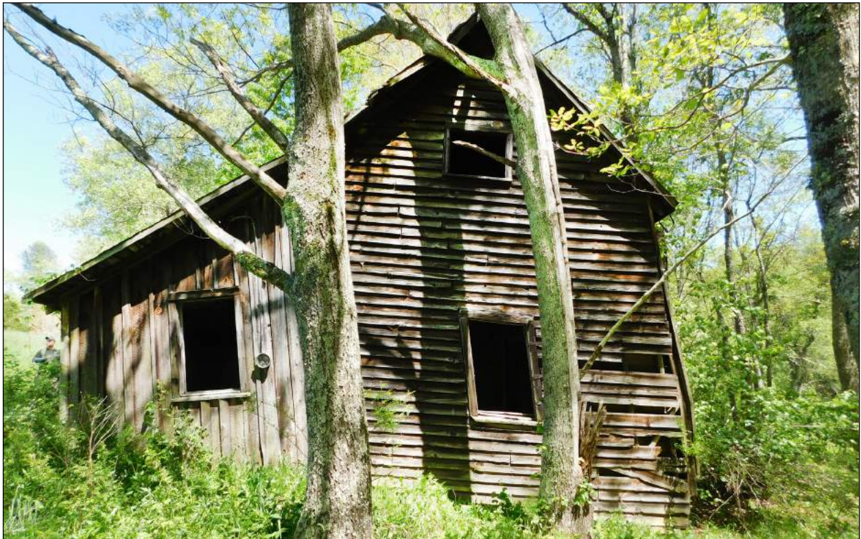
B. West Facing Side of House
