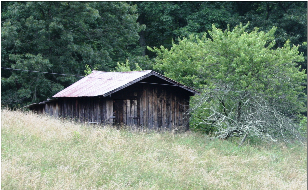
Figure 10. 035-5136, Crib Barn #1. Photo taken 23 June 2017, facing northeast.
