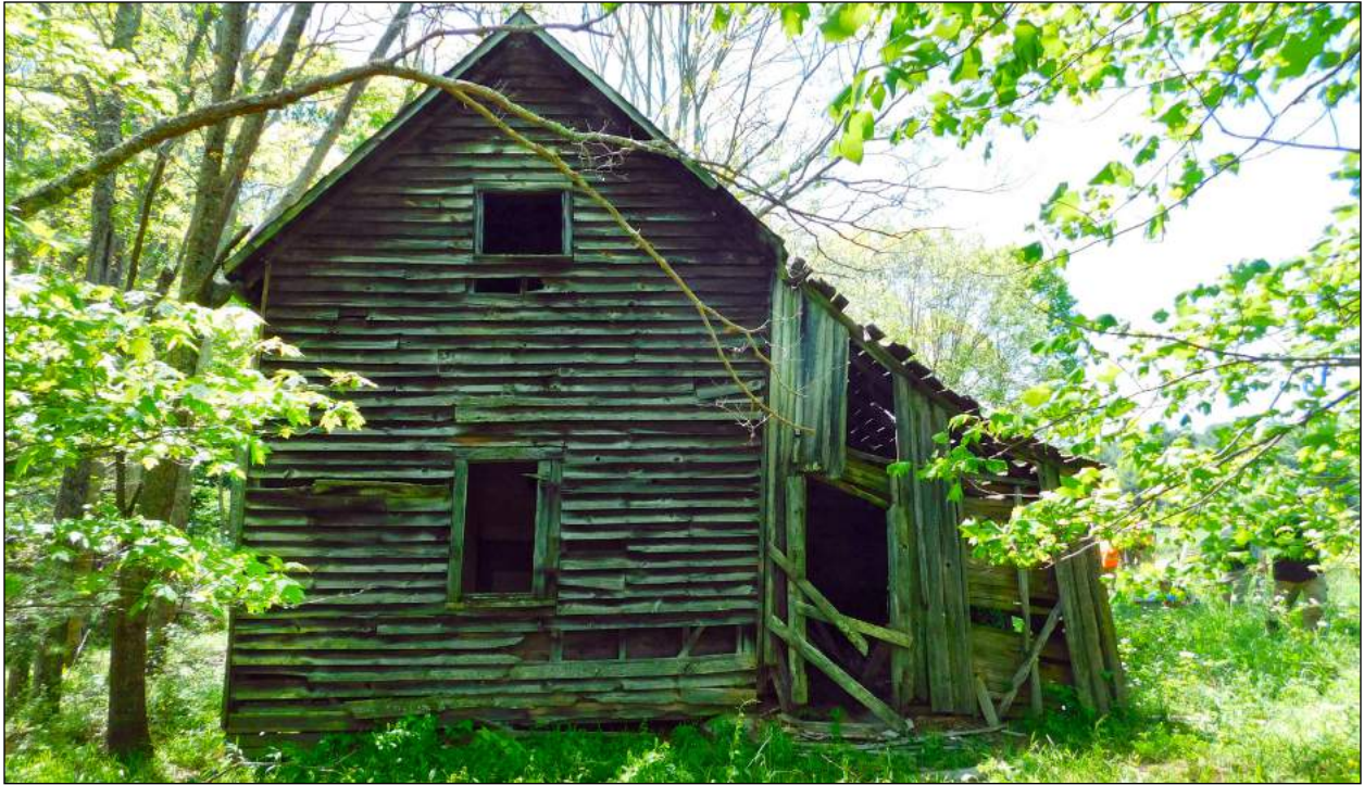
A. South Facing Side of House
