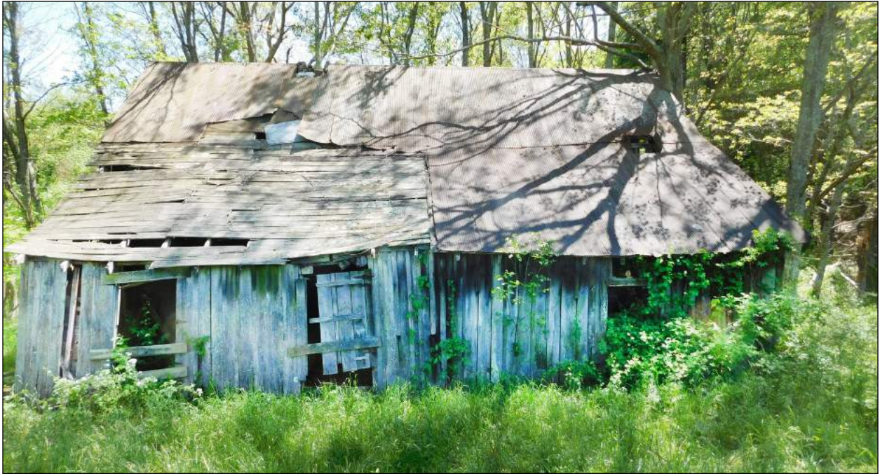
A. North Facing Side of House
