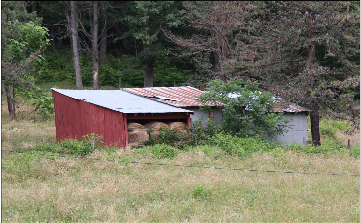
Figure 11. 035-5136, Crib Barn #2. Photo taken 23 June 2017, facing north.
