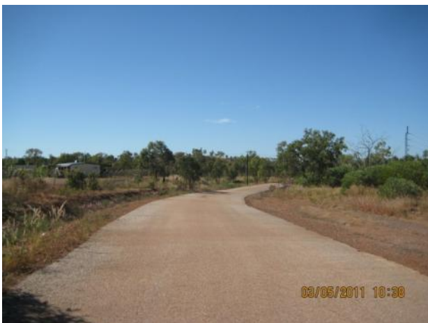
Figure 9 Internal Mine Roads, sealed section of roads
