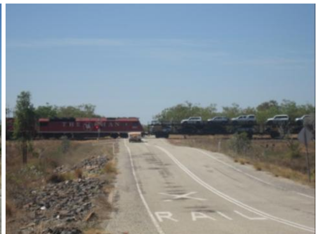
Figure 16 Edith Falls Road level crossing, view to east of flashing lights and on-road warning signage
