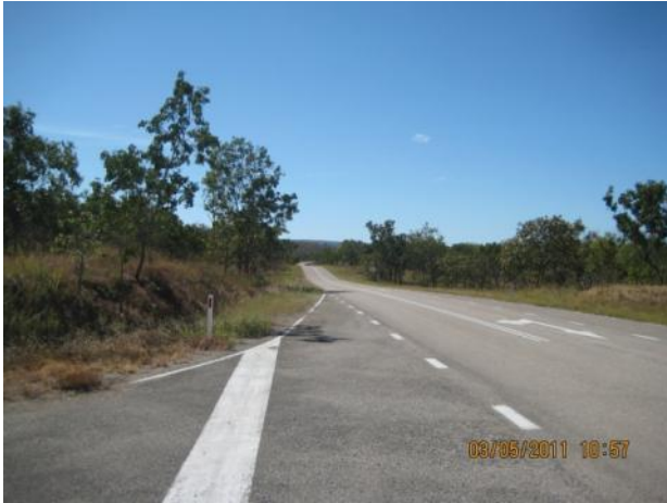
Figure 13 Sight distances at the Edith Falls Road / Jatbula Road (Mine Access Road) intersection, view to east on Edith Falls Road
