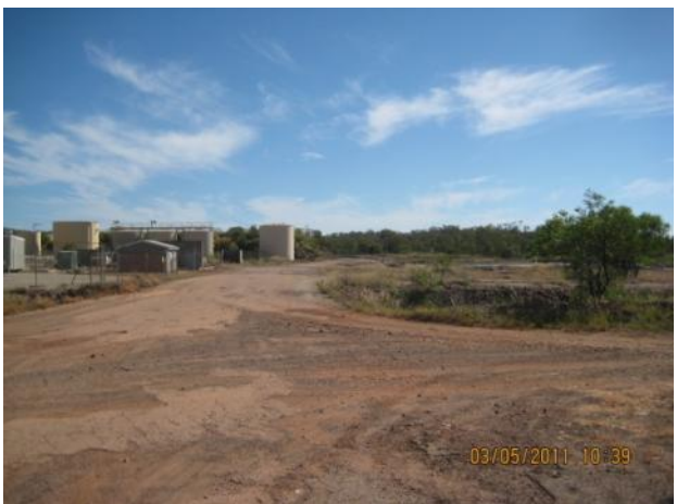
Figure 10 Internal Mine Roads, unsealed sections of roads
