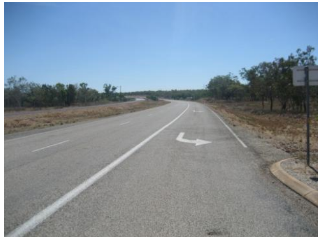
Figure 12 Sight distances at the Stuart Highway / Edith Falls Road intersection, view to north on Stuart Highway
