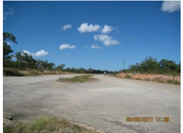
Figure 4 Stuart Highway dual carriageway cross section at Edith Falls Road intersection, view to south
