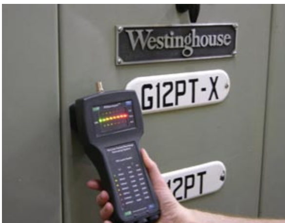
TEV Testing of Solid Insulated Switchgear
