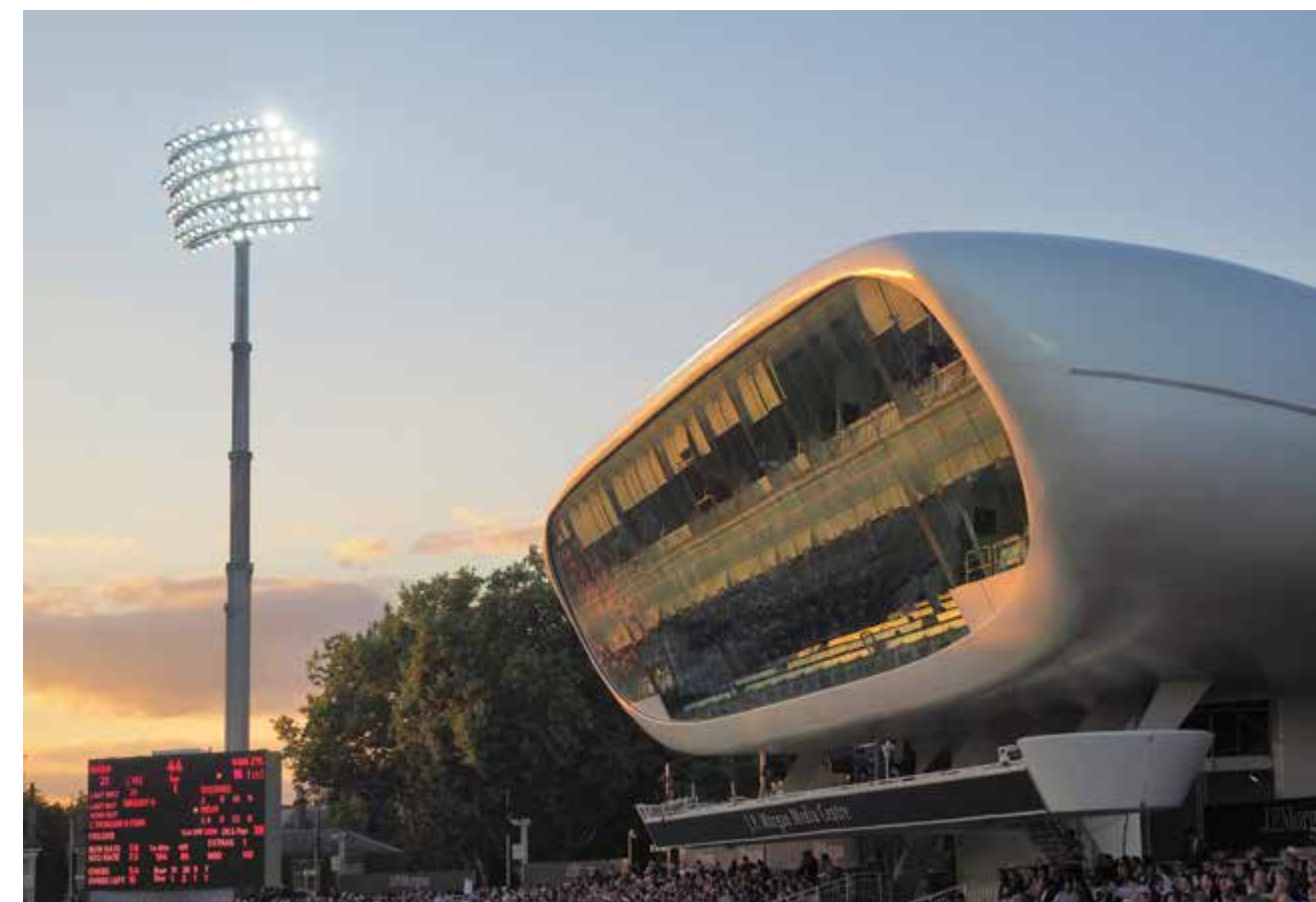
Lord's Cricket Ground Media Centre London, UK, 1999 Future Systems
