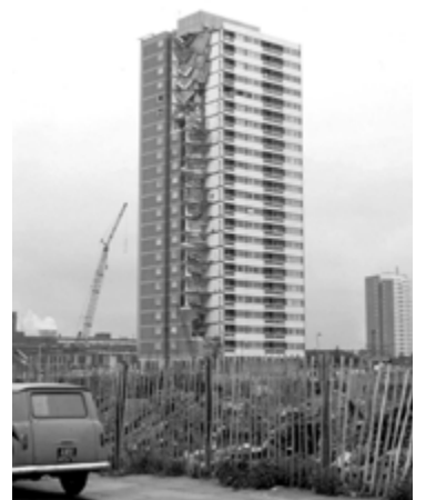
Ronan Point, London: construction started in 1966; it was demolished in 1968 following partial collapse after a gas explosion.
