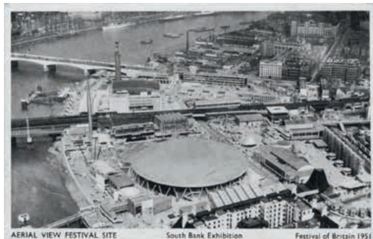
Above. Aerial view of the Festival of Britain site, showing the Dome of Discovery. London, UK, 1951
