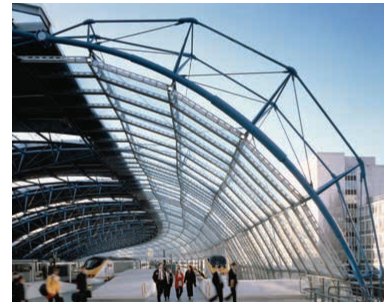
Above. International Terminal Waterloo London, UK, 1993 Nicholas Grimshaw & Partners/ Anthony Hunt Associates/ Cass Hayward & Partners/Tony Gee & Partners/ Red de Ferrocarriles Británicos
