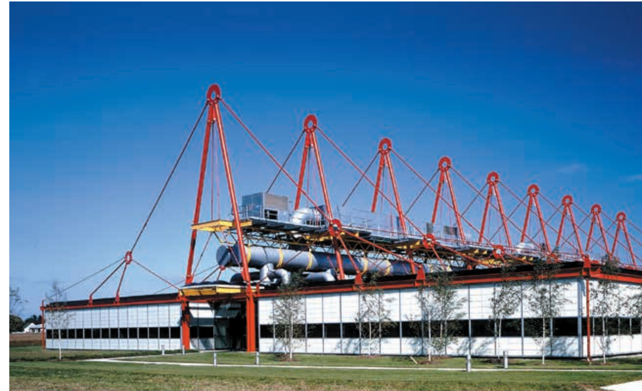
Left. PATMOS, Patscentre Princeton, USA, 1985 Richard Rogers Partnership, Kelbaugh and Lee Architects/ Ove Arup & Partners
