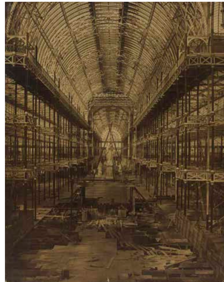
Right. The Crystal Palace being reconstructed at Sydenham London, UK, 1854. Originally constructed 1851, rebuilt 1854, destroyed 1936. Joseph Paxton/William Cubitt (engineer), Fox, Henderson & Co. (building contractors)
