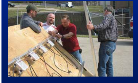
Figure 72. AC modules and micro inverters are small inverters installed integral to or adjacent to individual PV modules.
