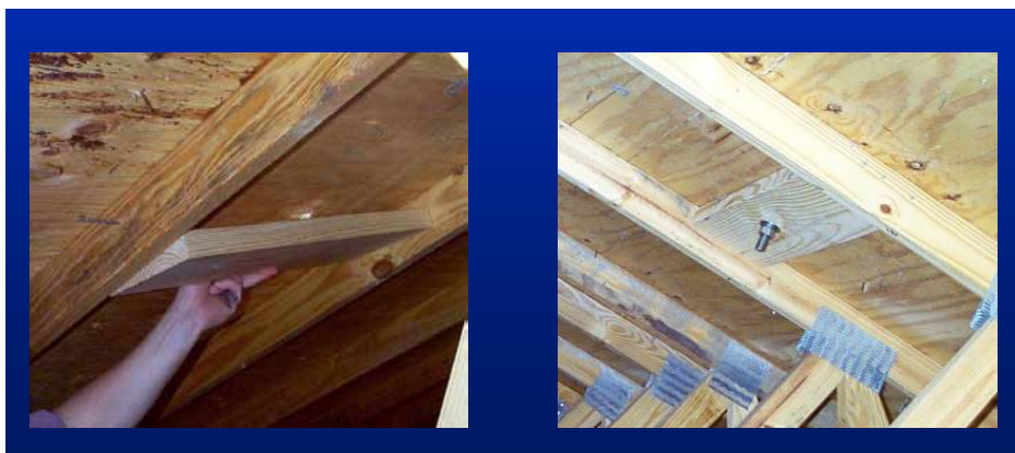
Figure 106. Additional blocking may be required for some installations to adequately secure point attachments to the structure.
