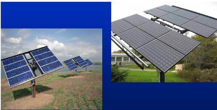
Figure 24. Sun-tracking arrays are typically mounted on poles and increase the amount of solar energy received.
