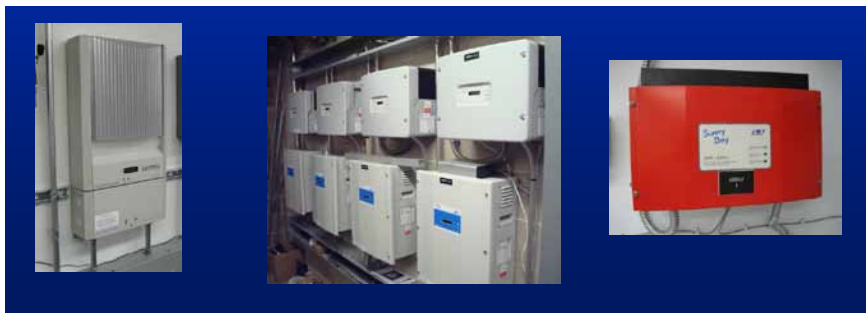
Figure 73. String inverters are small inverters in the 1 to 12 kW size range, intended for residential and small commercial applications.
