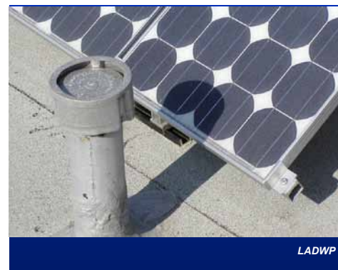
Figure 17. Shading of PV arrays can be caused by any obstructions interfering with the solar window.
