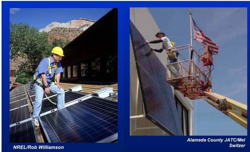
Figure 84. Fall protection is a primary safety concern for PV installers.
