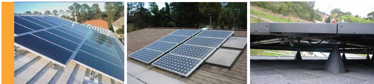
Figure 21. Standoff mounts are the most common way PV arrays are attached to sloped rooftops.
