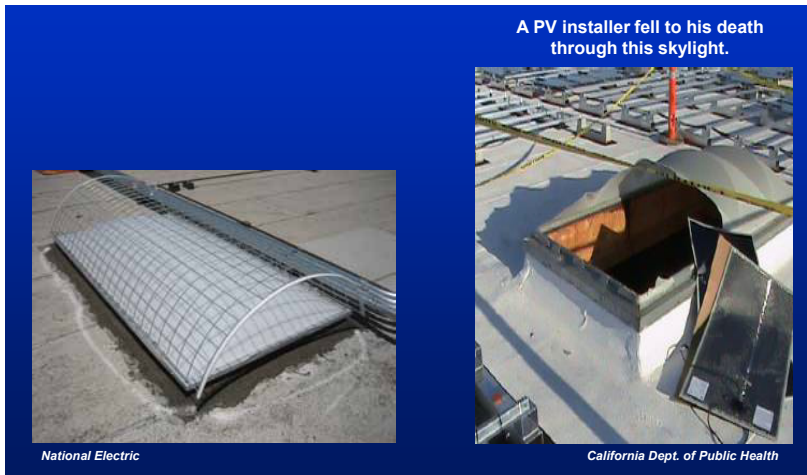
Figure 85. Skylights must be protected from fall hazards by barriers or covers.
