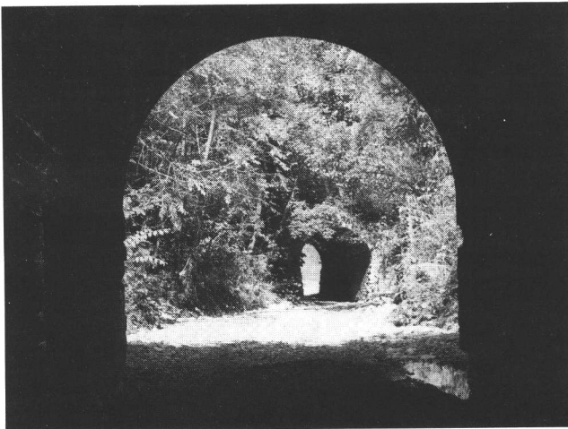
Fig. 15.—Culverts constructed of local limestone near Pearl, Pike County. These culverts supply the name—Twin Culvert Cave—for the nearby cave. An infrequently used county road and a small stream share the culverts.
