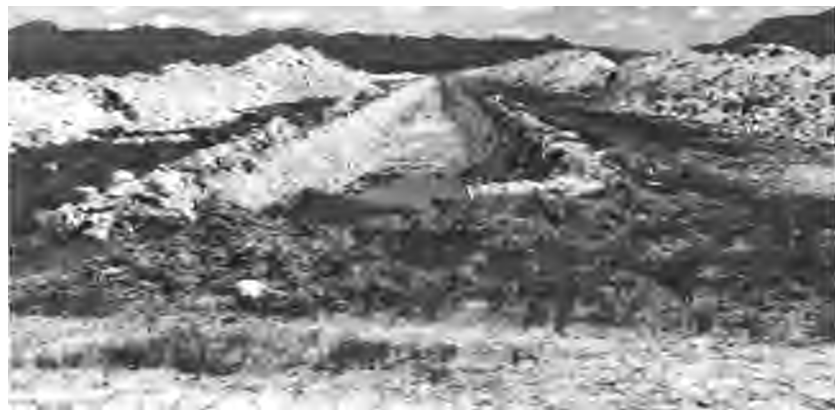
Figure 23. "New Canal," under construction (F18). View is east-northeast. August 1960.
