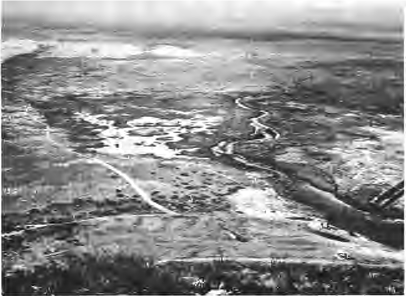
Figure 16. Posos de la Becerra ( SW\frac{1}{4} , 112), three days after completion of the drainage canal to the right; all the outflow marshes, center and to the right, now are dry. View is east. December 1964.
