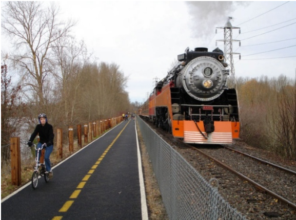
A popular RWT showing 8.5' minimum setback from edge of trail to rail centerline
