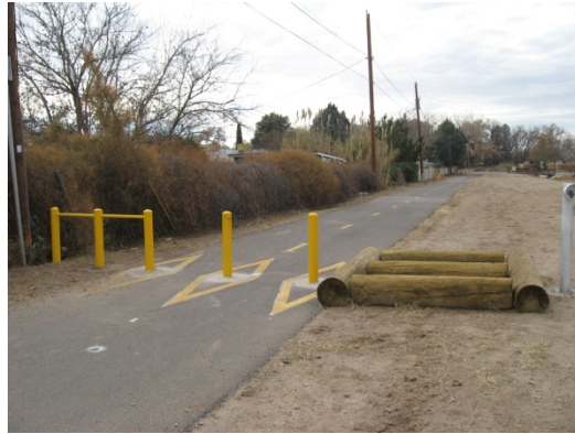
A combination of bollards, fencing and a "step over" were used on this trail to manage motorized access.
