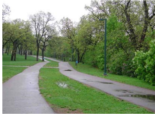
These split trails separate pedestrians and bicyclists. Trail signage and pavement markings direct users to the appropriate trails.
