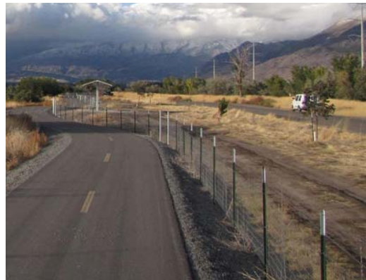
Fencing provides a physical barrier between the pathway and a parallel dirt road, keeping motorized vehicles off the trail.
