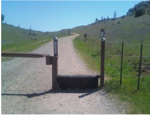
An equestrian caveletti, used in combination with fencing and a gate, deters motorized vehicles.
