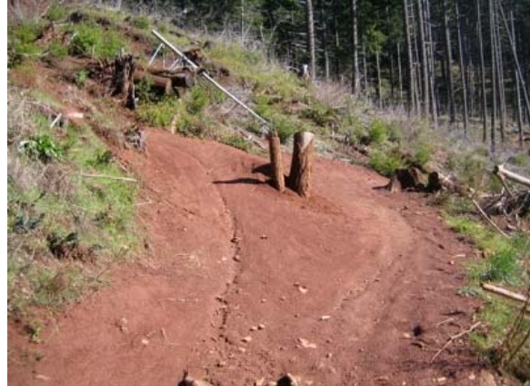
Natural surface trails are subject to erosion when water is allowed to travel along their length.
