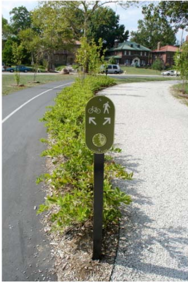
Vegetation, different surface treatments and signs assist users in choosing the appropriate pathway.
