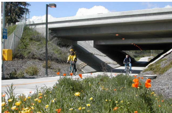
Type 4 grade-separated undercrossing
