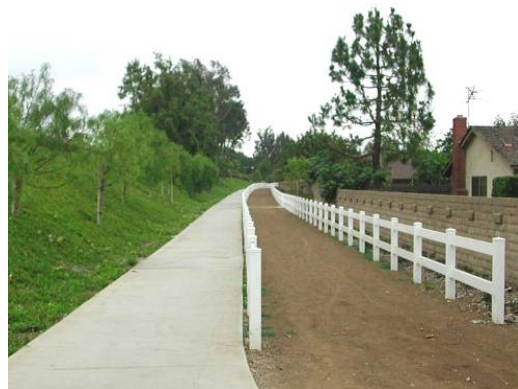
Fencing helps define the trail corridor. Pedestrians and bicyclists on the left, equestrians on the right.
