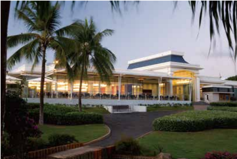
Club House overview with NIPPO Seamlessline lighting
