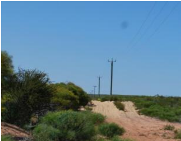
Photograph 7 – View of Western Power main transmission line to Kalbarri townsite.
