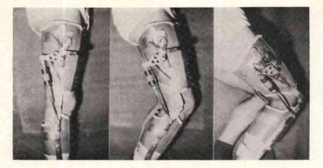
chanical principle of the connecting rod as was used for this particular case. The involuntary flexion of the patient's knee was brought to an "elastic stop" at a flexion angle of 145 degrees and injury of the knee prevented. A lever could be triggered to accomplish full knee flexion.
