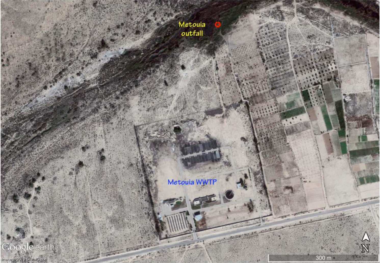
Map 76 Metouia/Ouethref WWTP and outfall (detailed view)
