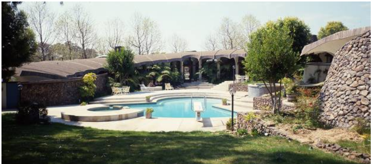
The Atoll residence designed by Kendrick Kellogg in 1972. Note the curvilinear roof form which mimics the site topography and the natural materials. Courtesy of Keith York.
