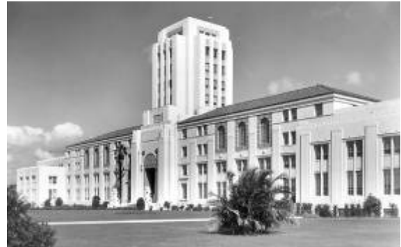
The San Diego Civic Center, now known as the County Administration Center, 1936-38. Courtesy of the San Diego Historical Society.
