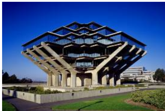
UCSD Geisel Library designed by William Pereira in 1970. Note the heavy concrete base with striking angles, repeated forms, and glass top. Courtesy of UCSD.
