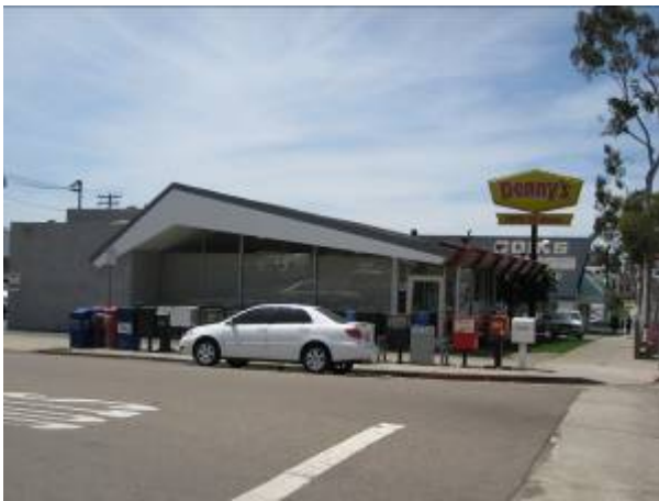
Denny's Restaurant on El Cajon Blvd., designed by Arnett & Davis. Note the boomerang roofline, prominent signage, and large aluminum framed windows.
