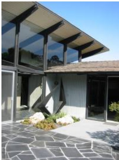
The Mills residence in La Jolla, designed by Dale Naegle in 1957. Note the scissor rafters in the entry foyer and the dramatic full-height glass. The arrangement of the floor plan around a central courtyard and the continuous interior/exterior flooring add to the strong outdoor connection.
