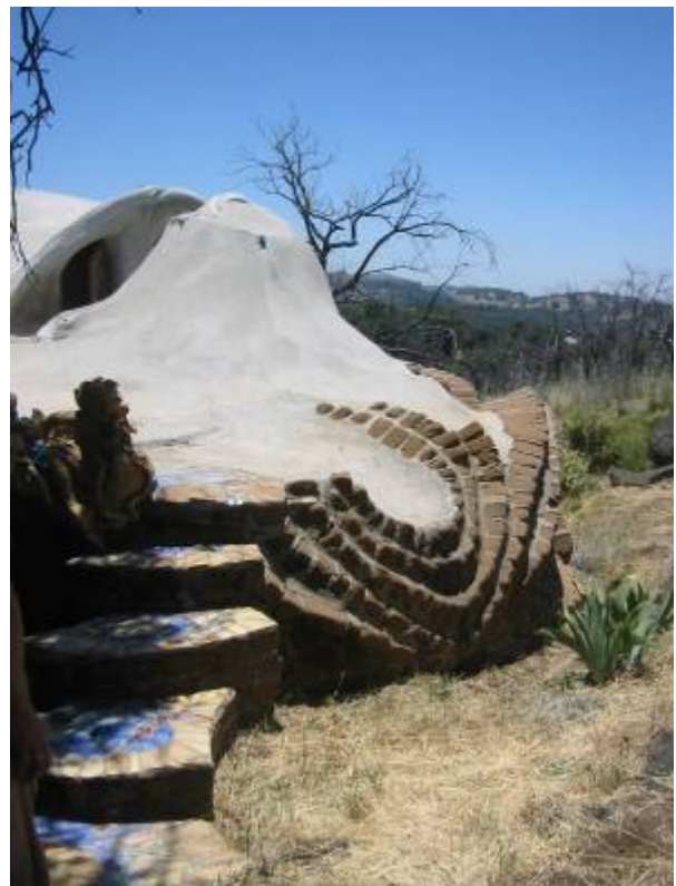
The "Boys House" at the Hubbell Compound, Note the mix of materials including plaster, adobe, stone, and tile. The structures are sculptural in form and every detail has been considered in the design.
