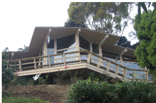
Silva Residence in Point Loma, by Sim Bruce Richards, 1953. Note the wide eaves and exposed beams. Large windows and a deck both exhibit a pointed, triangular, orientation. The large deck overhang leaves the natural slope of the site untouched.
