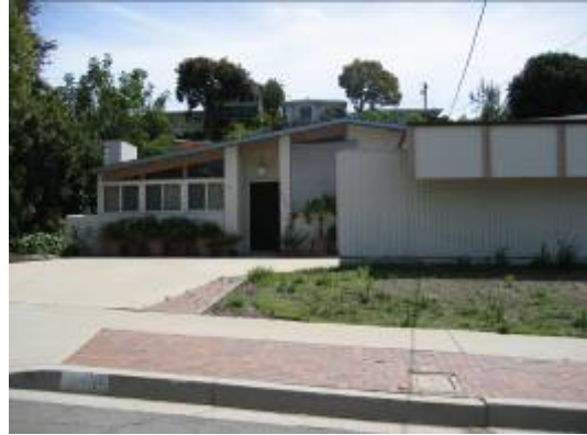
Contemporary tract home design by Palmer and Krisel for Drogin Homes ca. 1960. The same floor plan is used throughout this neighborhood with variations to the roofline.
