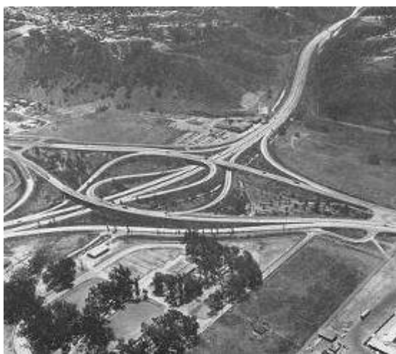
Highway 395 and 80 (now Highway 163 and Interstate 8) Mission Valley interchange, 1948. Courtesy of California Highway and Public Works.
