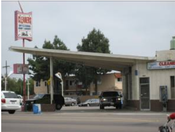
Commercial building on El Cajon Blvd. This roof form is common in gas stations and drive-thrus from this era, also note the prominent signage.
