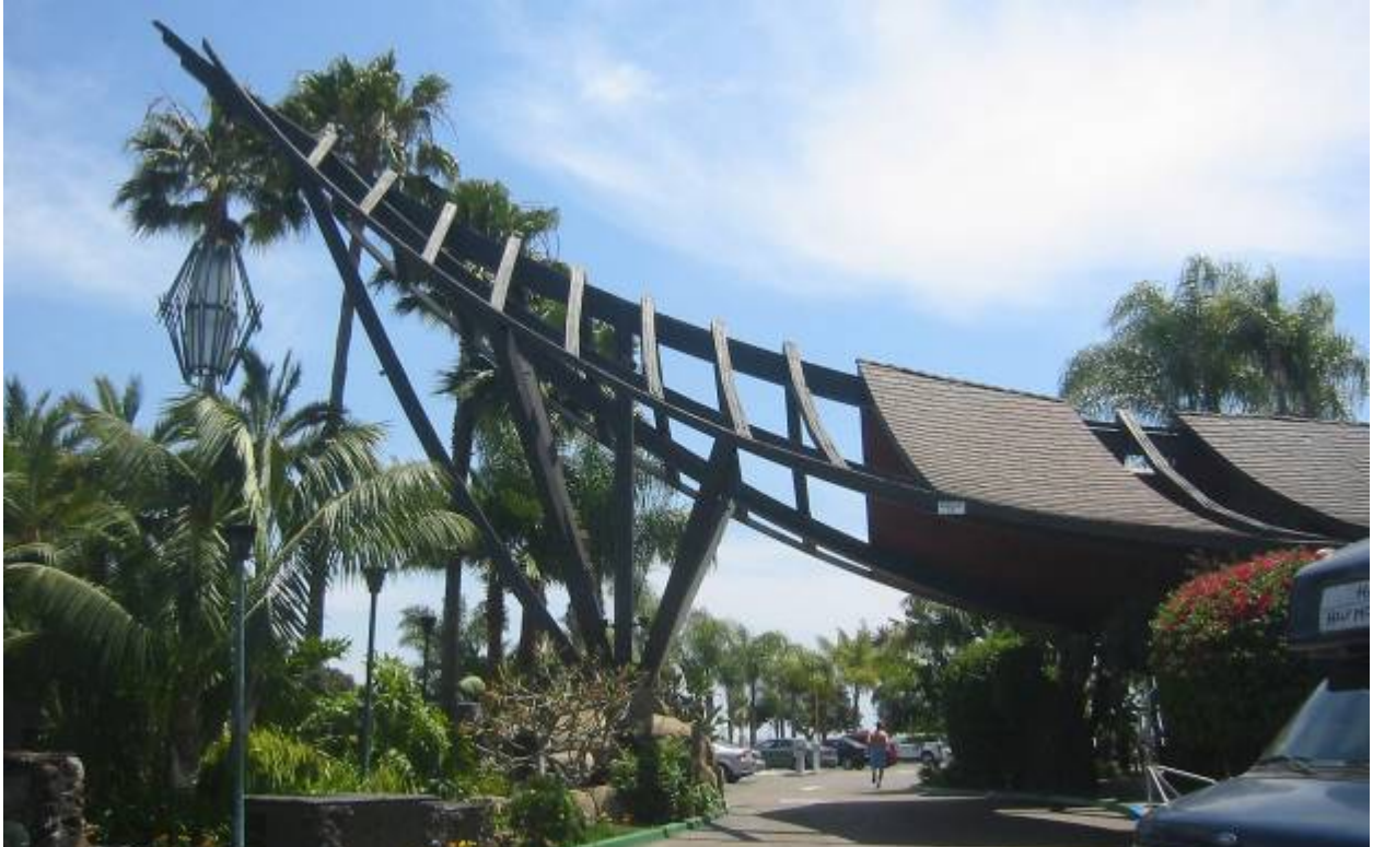
Humphrey's Half Moon Inn at Shelter Island, designed by Hiram Hudson Benedict in 1965. Note the dramatic cross-gabled porte-cochere with the massive curved ridge beam which is accentuated by the selective absence of roofing. This building also features a lush tropical landscape and a decorative lantern at the tip of the roof. The entire structure is reminiscent of a boat hull.
