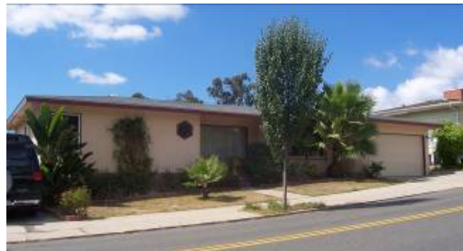
This example of a Tract Ranch style house in Rolando exhibits character defining features such as a low-pitch hipped roof, stucco exterior finish, low horizontal massing and attached two car garage. Note the Moderne inspired window design including a corner window and small hexagonal window.
