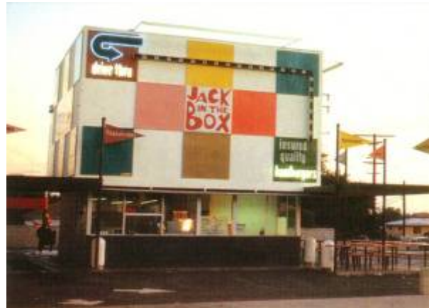
Jack-in-the-Box restaurant, Mission Hills, designed by Russell Forester, ca. 1950s. The building epitomizes the building as billboard concept. Courtesy of Jack-in-the-Box archives.
