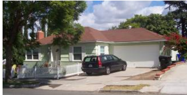
Located in Rolando, this Tract Ranch residence exemplifies mixing of traditional architectural details such as horizontal wood siding, wood shutters and a brick chimney with modern conveniences such as the attached two car garage..
