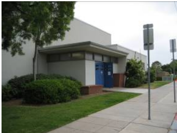
McKinley Elementary School in North Park, designed by Richard Requa, ca. 1937. Note the stucco façade with brick skirt, the horizontal arrangement of windows, the flat roof, and vertical projection marking the front entry.
