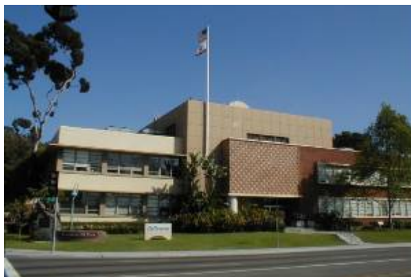
Caltrans building in Old Town, designed by CJ Paderewski in 1953. Note the horizontal bands of windows accented by a plaster surround.
