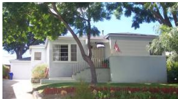
This Minimal Traditional residence located in Rolando features a combination of stucco and wood siding exterior finish materials, Moderne inspired corner windows and a detached rear garage.
