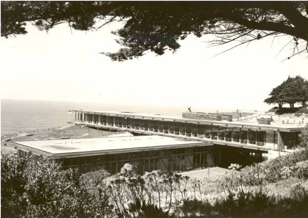
The Institute of Geo-Planetary Physics at the Scripps Institution of Oceanography in La Jolla, designed by Lloyd Ruocco in 1963. The post-and-beam construction allows for continuous floor-to-ceiling glass. The horizontal lines are accentuated by sun trellises and catwalks that encircle the building. The landscape was designed by Harriett Wimmer. Courtesy of the San Diego Historical Society.
