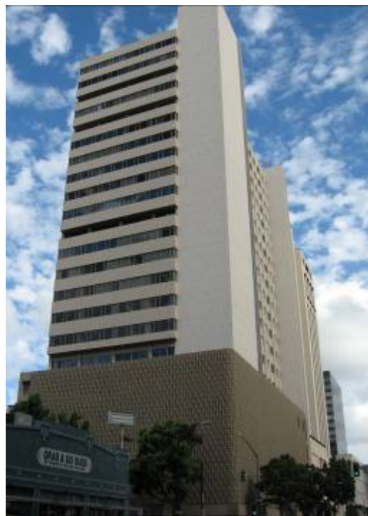
The Chamber Building in downtown San Diego, by Palmer & Krisel dates from 1963, and exhibits International style design elements inspired by the PSFS building in Philadelphia.
