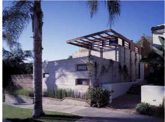
Rudolph Schindler's Pueblo Ribera Court, 1923. Schindler's slipform concrete construction technique resulted in the visible horizontal lines in the wall plane. Courtesy www.mosslerdoe.com .
