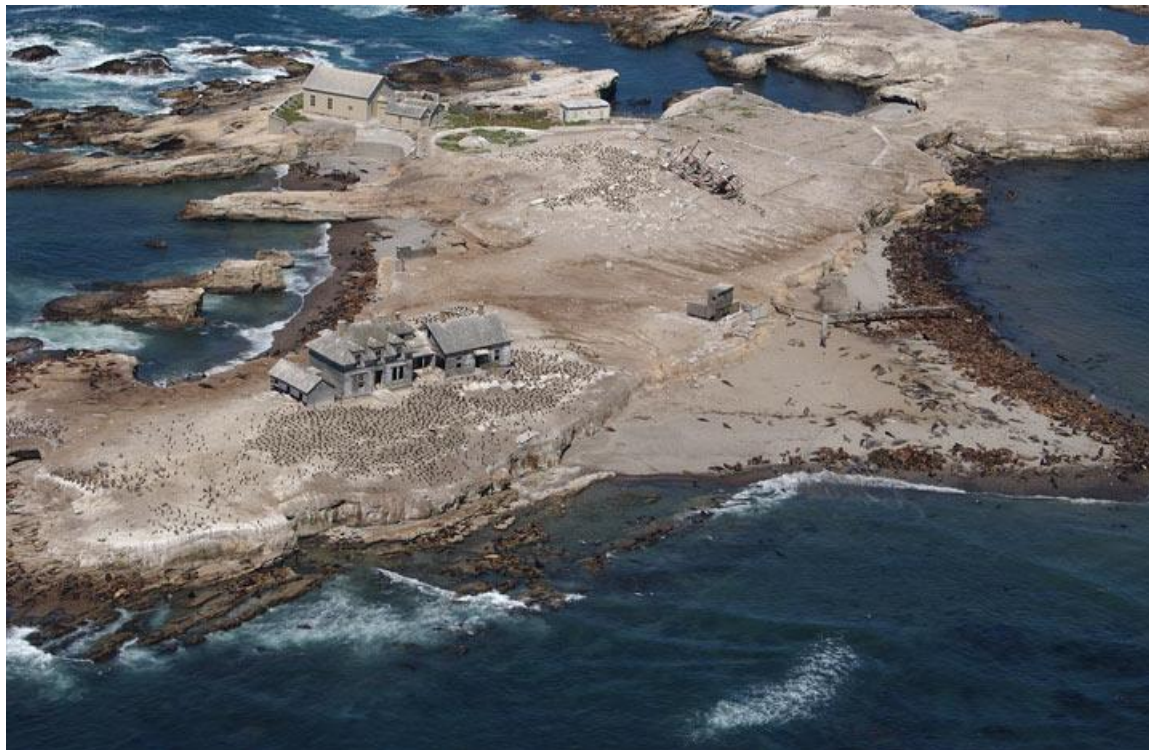
Año Nuevo Island. Lighthouse keeper's house in the foreground, refurbished fog signal and fuel storage buildings in the rear.
