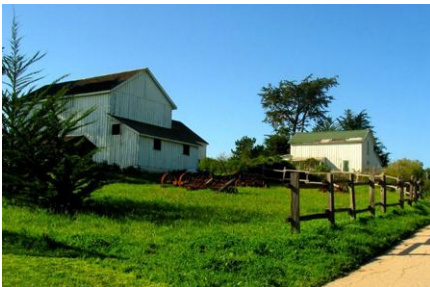
Dickerman dairy barn, left, and rear of Dickerman-Steele-Elliott house, right.
